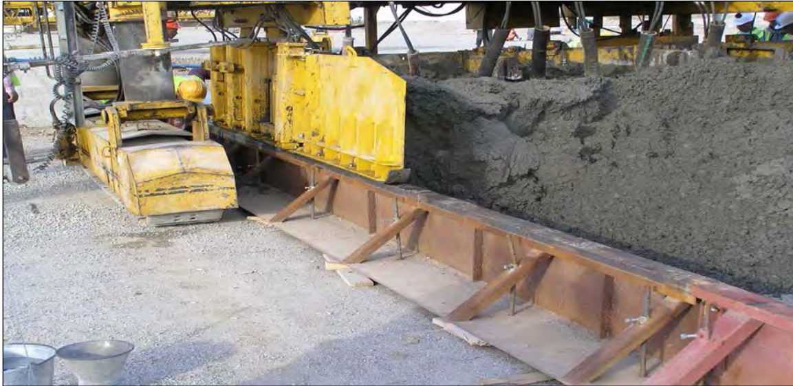
Figure 4-88 Slipform Paver Placing Concrete Inside Fixed Forms (Note Curved Skid Plate on Paver Mud Box. Also Note the Forms are Built Up With Cribbing. This is Unacceptable)
