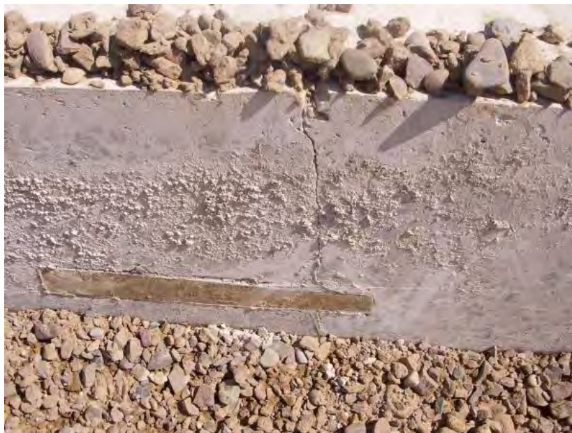
Figure 4-50 Misaligned Contract Joint Dowels
