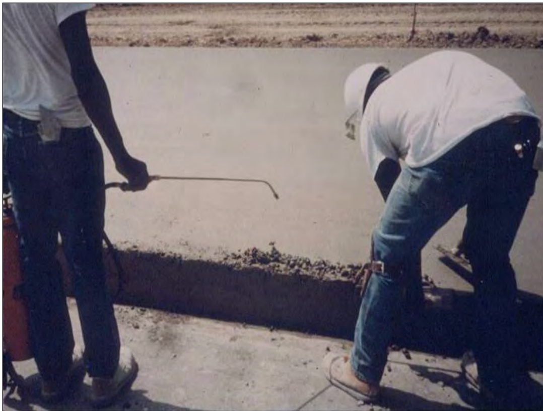
Figure 4-161 Over Finishing Edge of Pilot Lane
