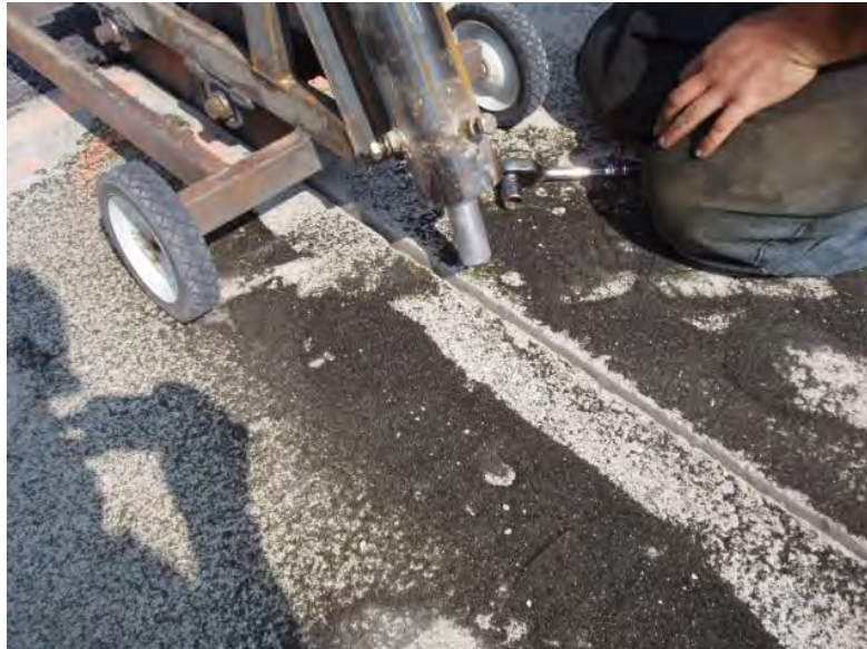
Figure 4-150 Sandblasting Joint
