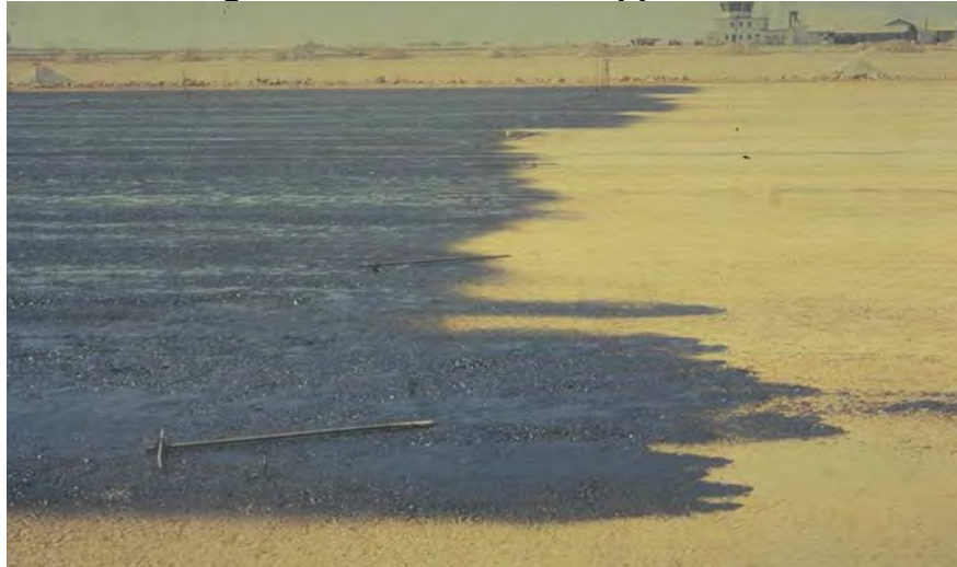
Figure 3-25 Prime Coat Application
