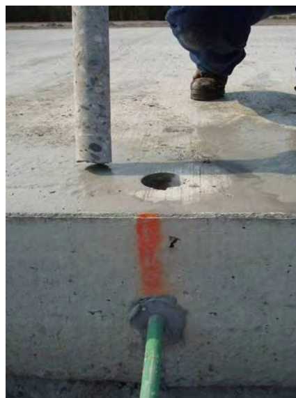
Figure 4-64 Cored Dowel to Verify the Grouting Technique
