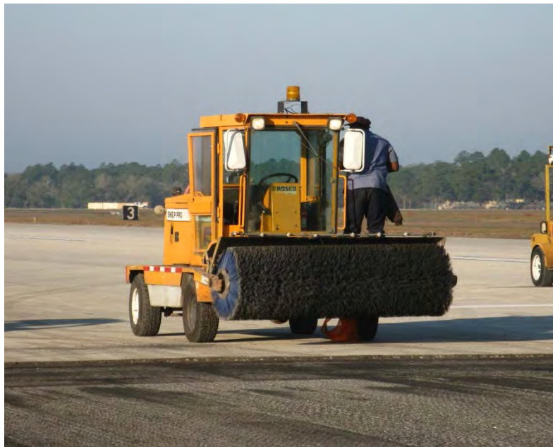
Figure 3-20 Sweeper for Cleaning Pavement Surface Prior to Tacking
