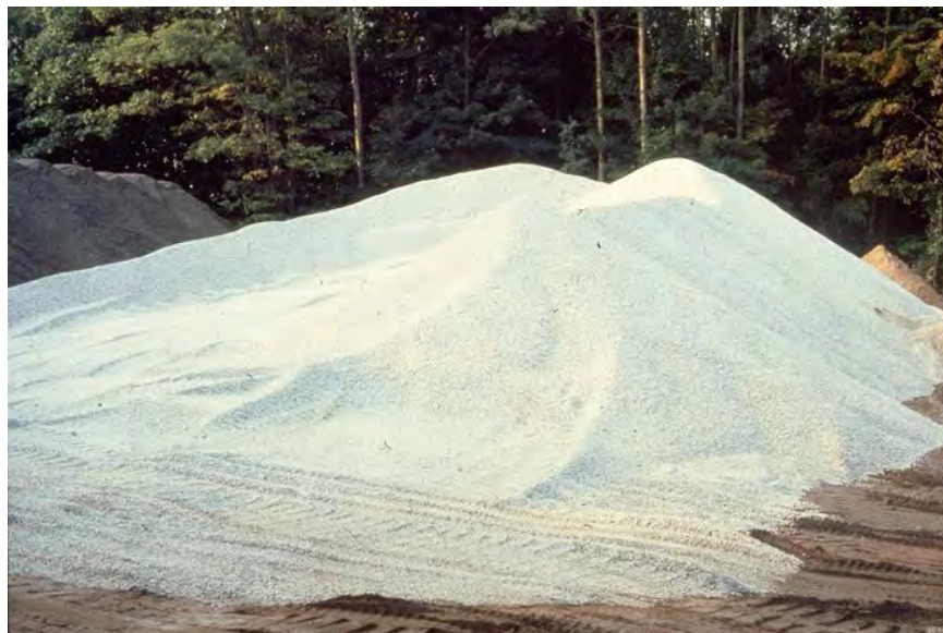
Figure 3-7 Stockpile Created on Sandy Surface
