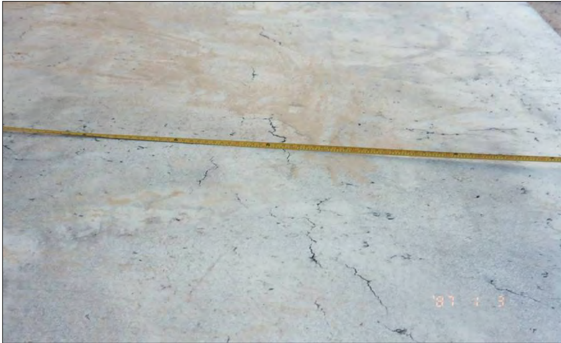
Figure 4-159 Plastic Shrinkage Cracking
