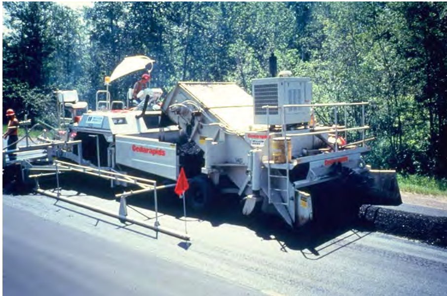
Figure 3-28 Dumping Directly into Paver
