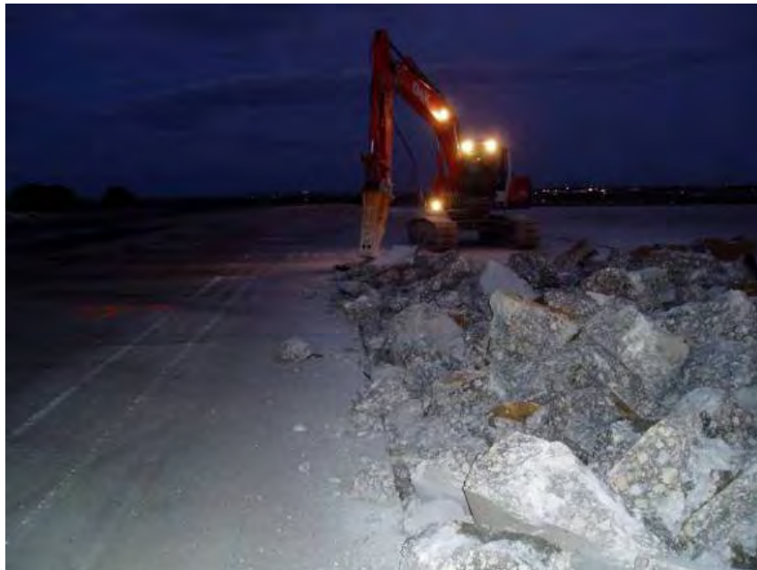
Figure 4-29 Demolition With No Protection of Adjacent Concrete
