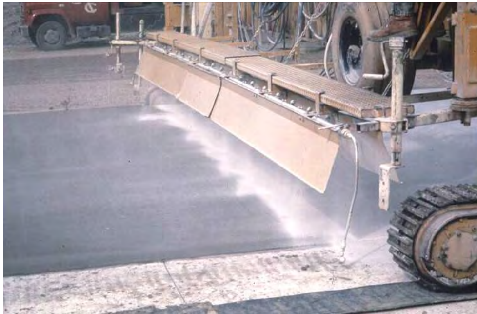
Figure 4-114 Good Application With Overlapping Spray and Windscreens
