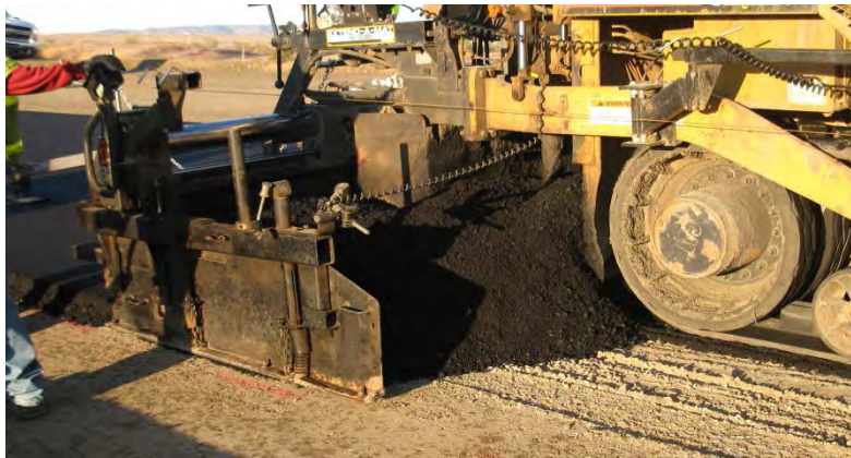
Figure 3-37. Excessive Distance between Auger and Side Plate
