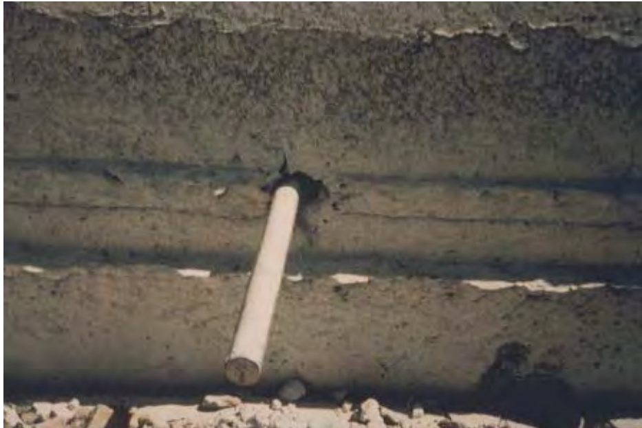
Figure 4-54 Voids around an Inserted Dowel
