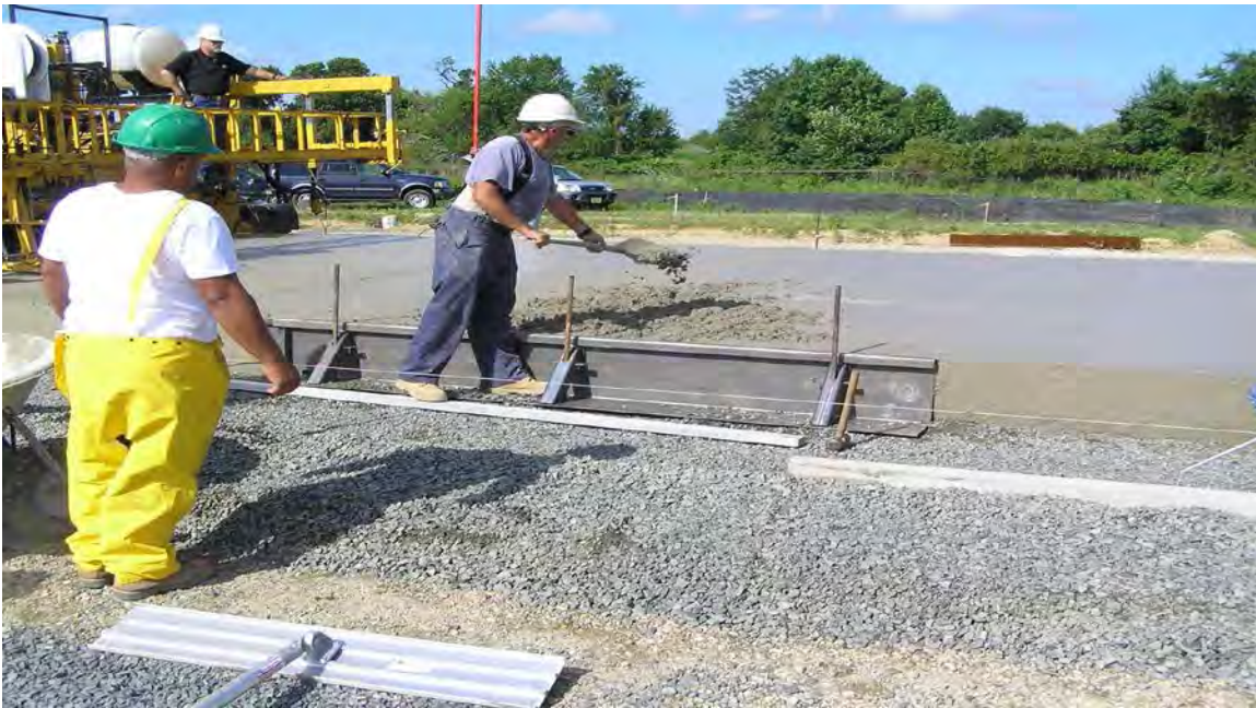
Figure 4-85 Acceptable Repair of Edge Slump
