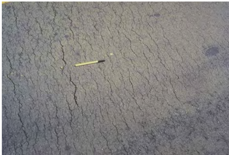
Figure 3-46 Checking Under Steel Wheel Rollers
