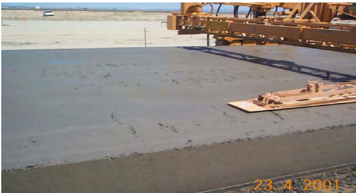
Figure 4-81 Poor Consolidation on Horizontal Surface of Slab
