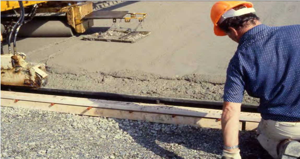
Figure 4-93 Excess Paste on Surface
