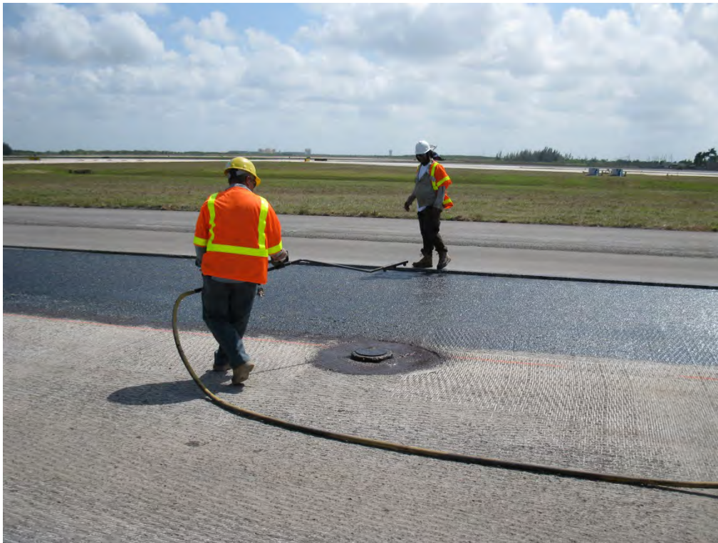
Figure 3-24 Application of Tack Coat with Hand Sprayer
