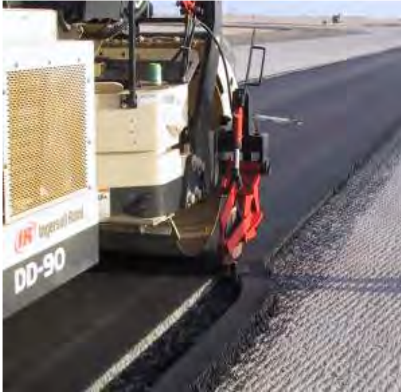
Figure 3-41 Use of Tapered Longitudinal Joint is not Desired
