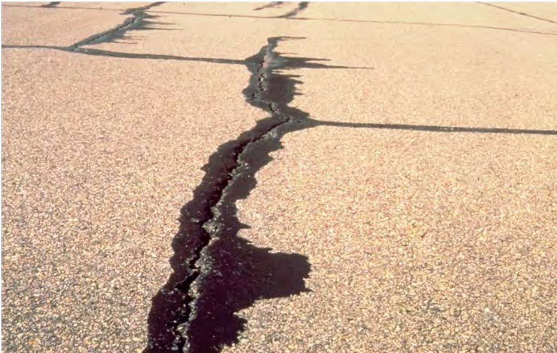
Figure 3-19 Excess Sealant
