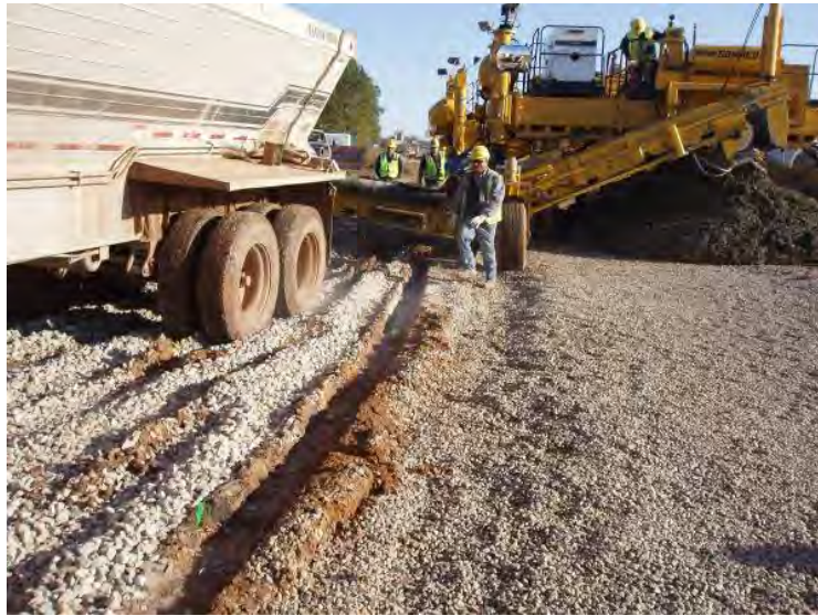
Figure 4-20 Disturbed Base Course from Equipment
