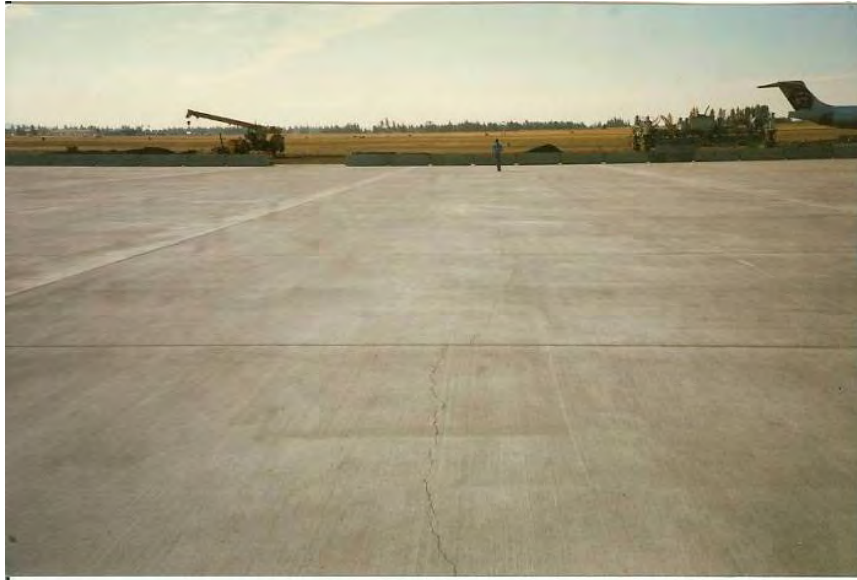
Figure 4-127 Mid-panel Cracking
