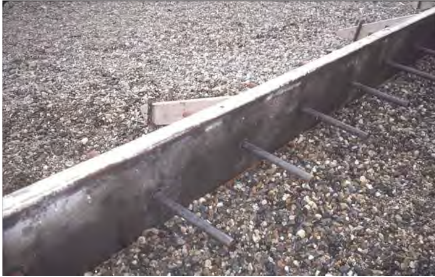
Figure 4-51 Dowels in Steel Forms
