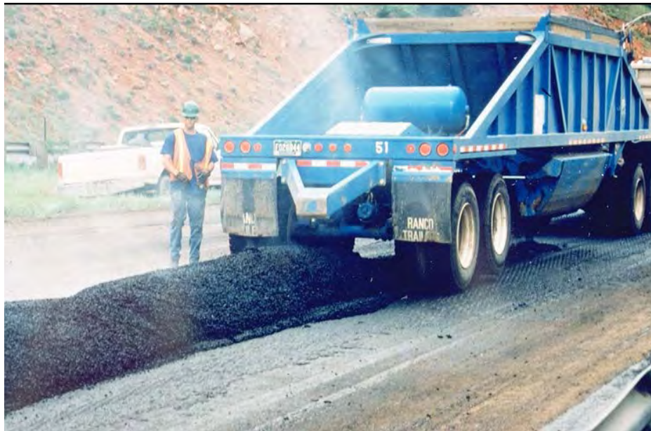
Figure 3-26 Placing of Windrow
