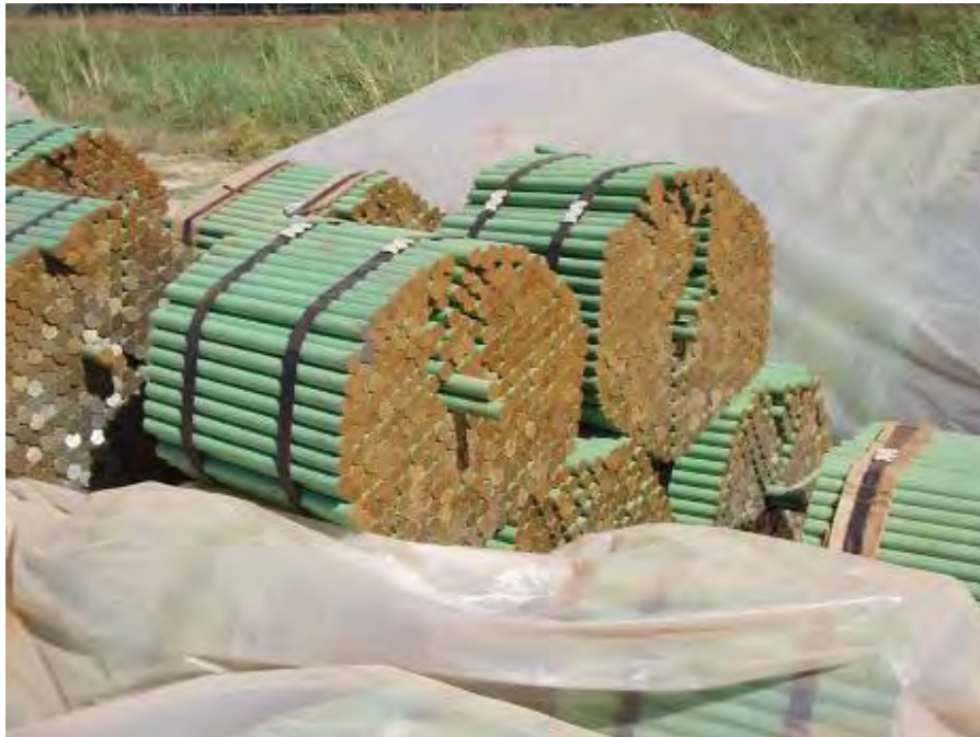
Figure 4-44 Dowels at Contraction Joints
