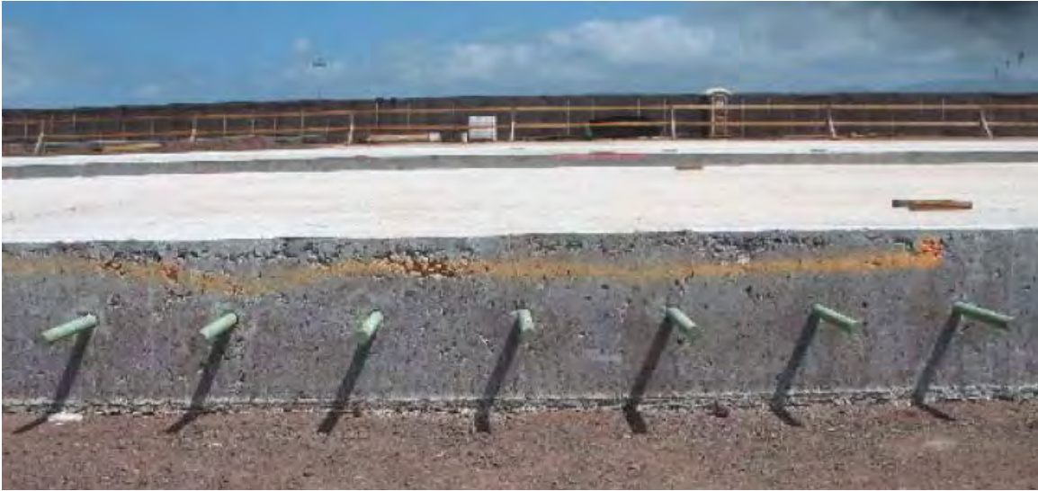
Figure 4-91 Unconsolidated Concrete Due to Lack of Vibration at Slab Edge
