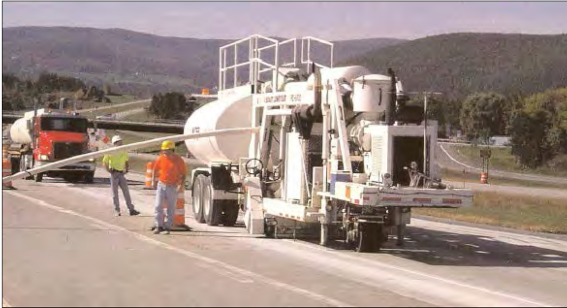
Figure 4-126 Diamond Grinding
