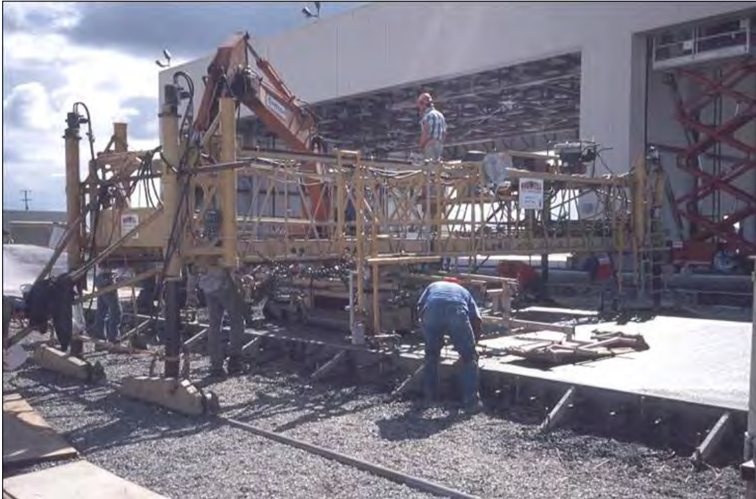
Figure 4-90 Truss-Mounted Paver and Carriage. Paver is Moving from right to left
