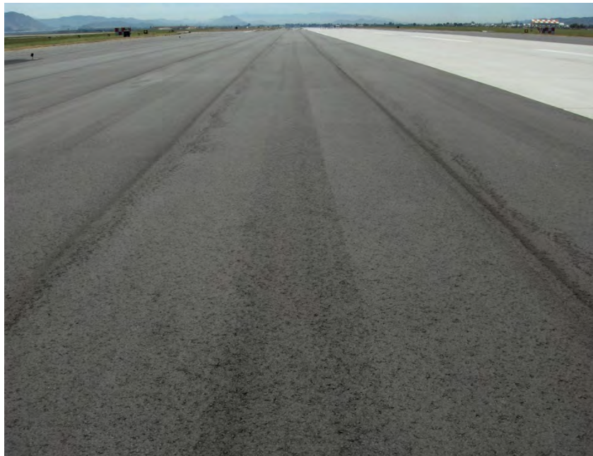
Figure 3-34 Uneven Surface after Compaction
