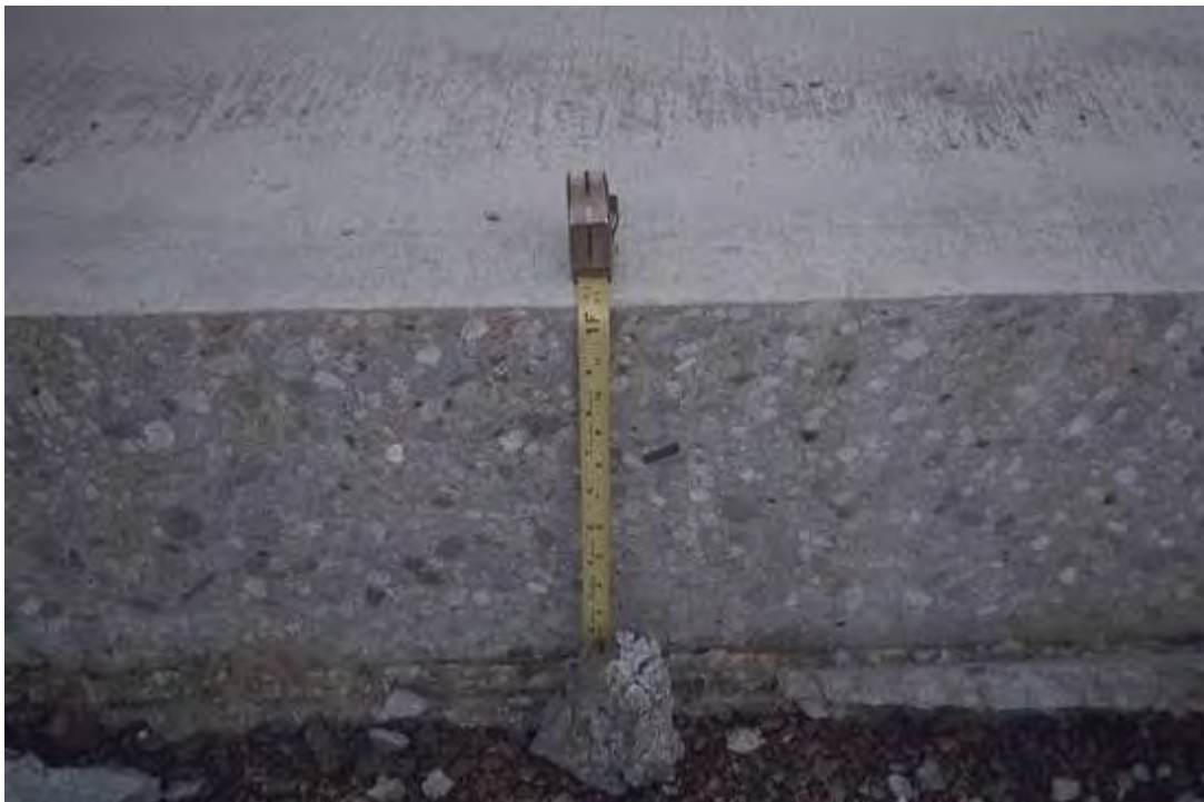
Figure 4-21 Full Depth Sawcut
