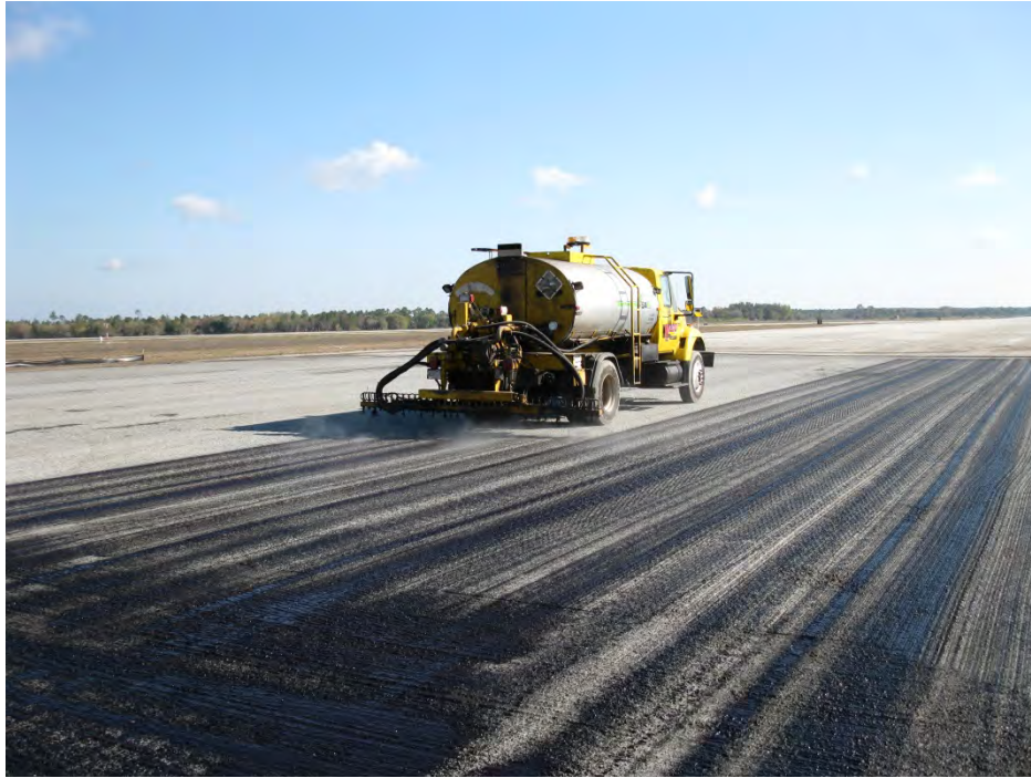
Figure 3-23 Excess amount of Tack Coat
