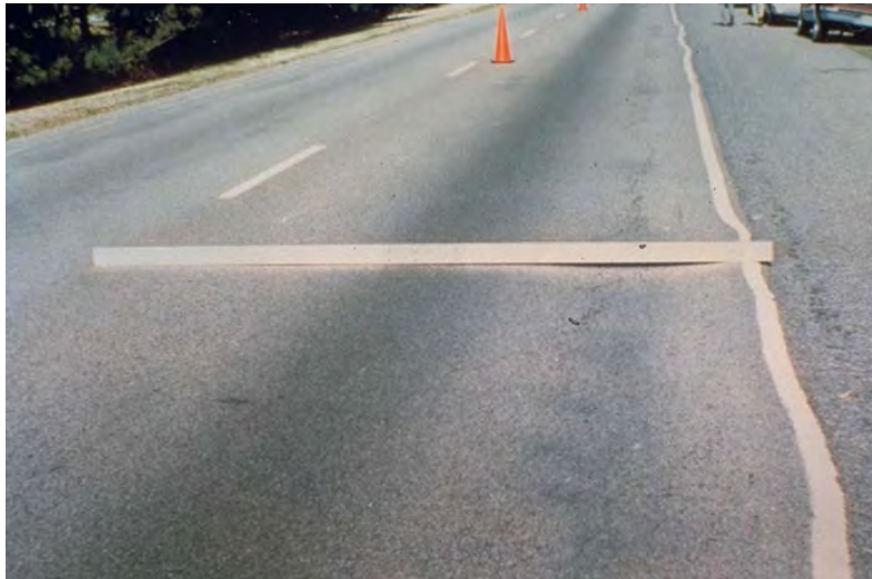
Figure 3-61 Block Cracking
