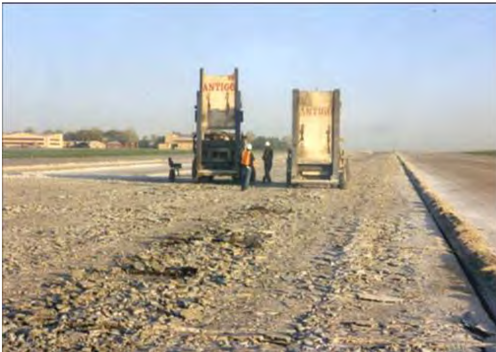
Figure 4-25 Improper removal Techniques - No Double Saw Cut
