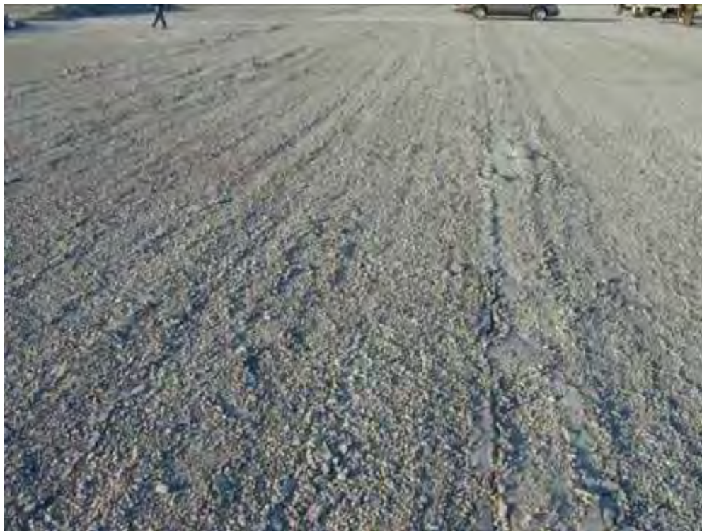
Figure 4-33 Rubblized Surface With The Resonant Rubblizing Technique
