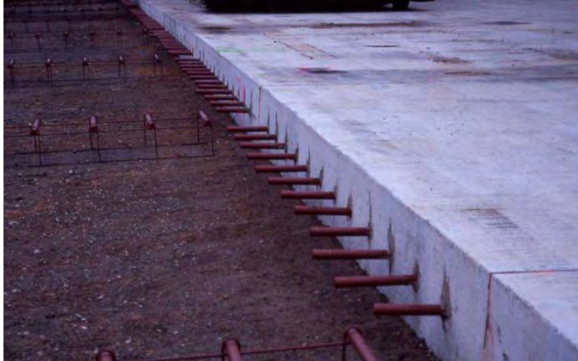
Figure 4-43 Dowel Ends not Epoxy Coated
