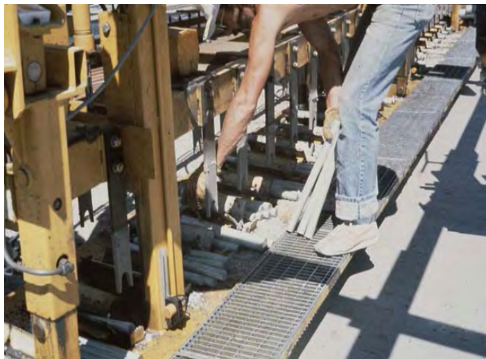
Figure 4-48 Inserting Contraction Joint Dowels – Slipform Construction
