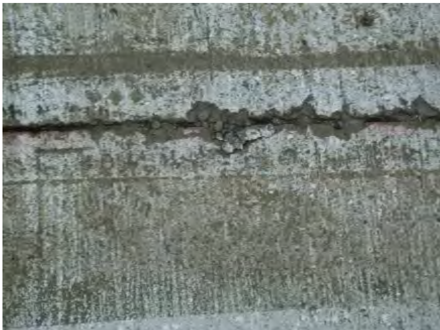
Figure 4-138 Spalling from Premature Saw Cutting
