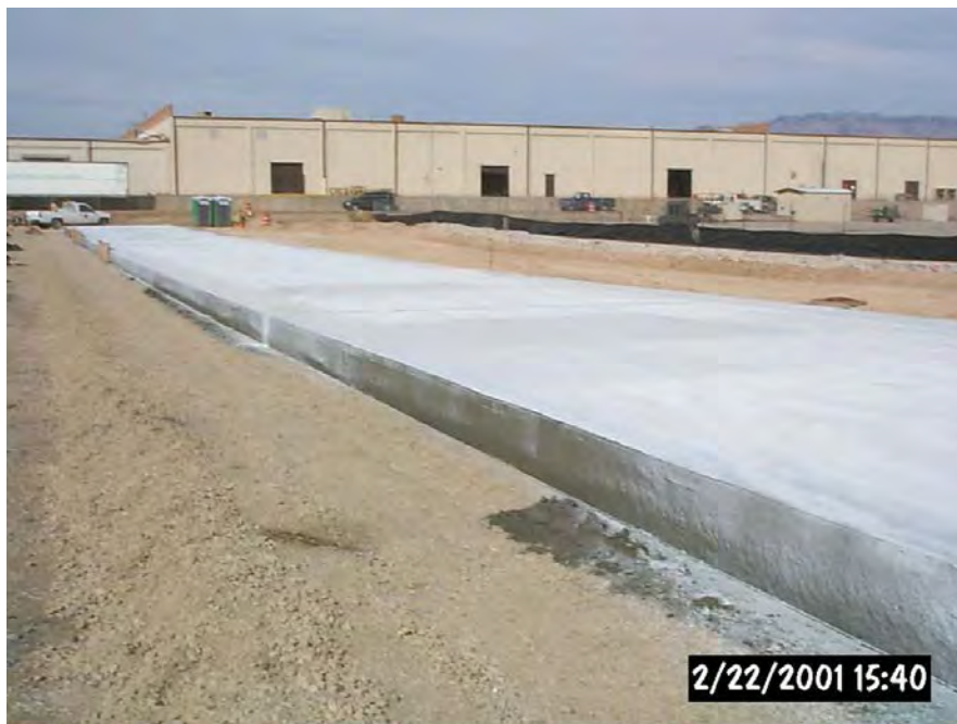
Figure 4-116 Poor Application of Curing Compound Vertical Joint
