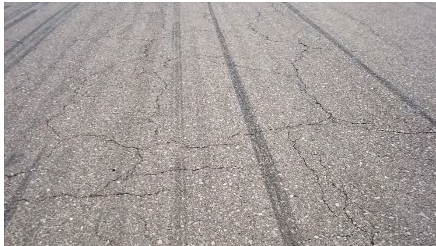
Figure 3-61 Block Cracking
