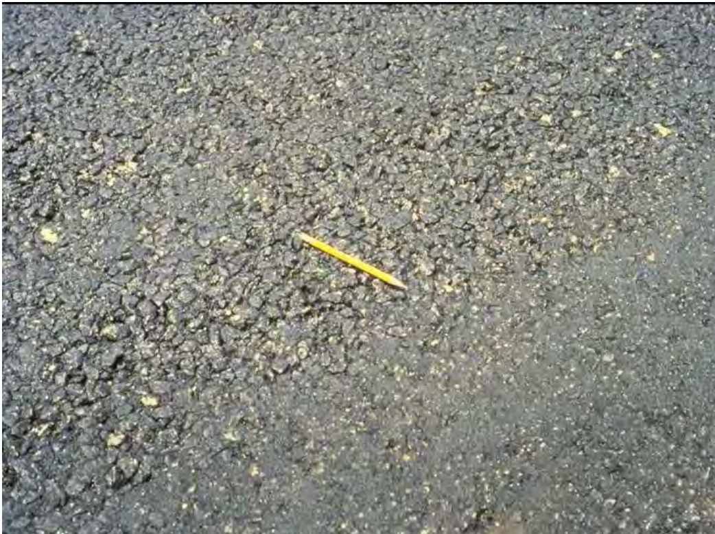
Figure 3-31 Segregation of Asphalt Mixture
