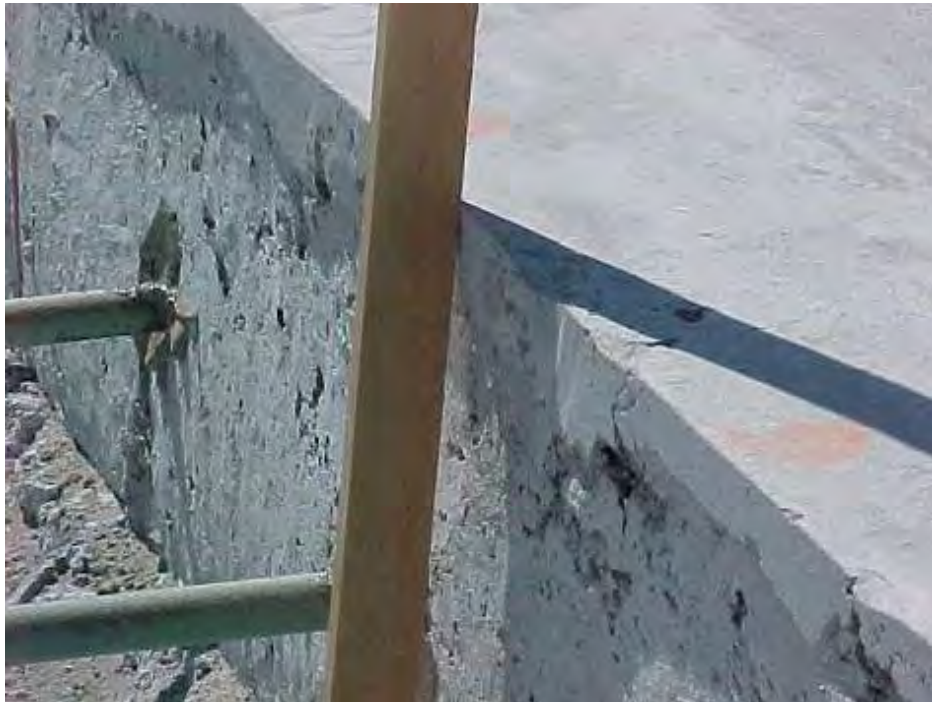
Figure 4-131 Out of Tolerance Joint Construction –Vertical Edge
