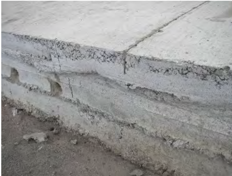
Figure 4-130 Poor Quality Thickened-Edge Joint Construction
