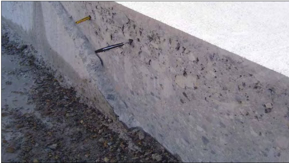
Figure 4-80 Poor Consolidation of Vertical Face of Slab
