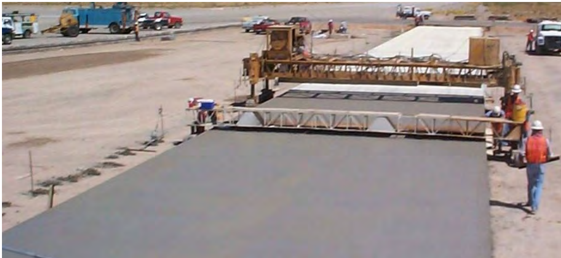
Figure 4-109 Burlap Drag Texture Applied From Hand Operated Bridge.
