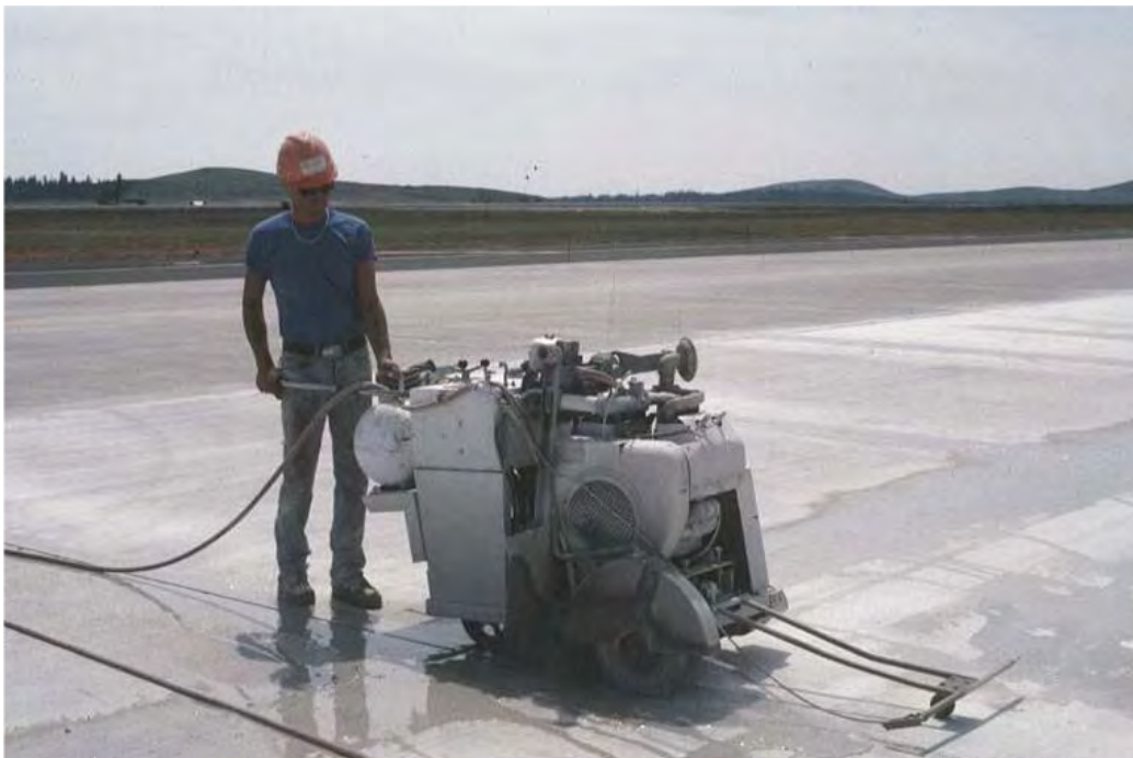
Figure 4-139 Early Entry Saw
