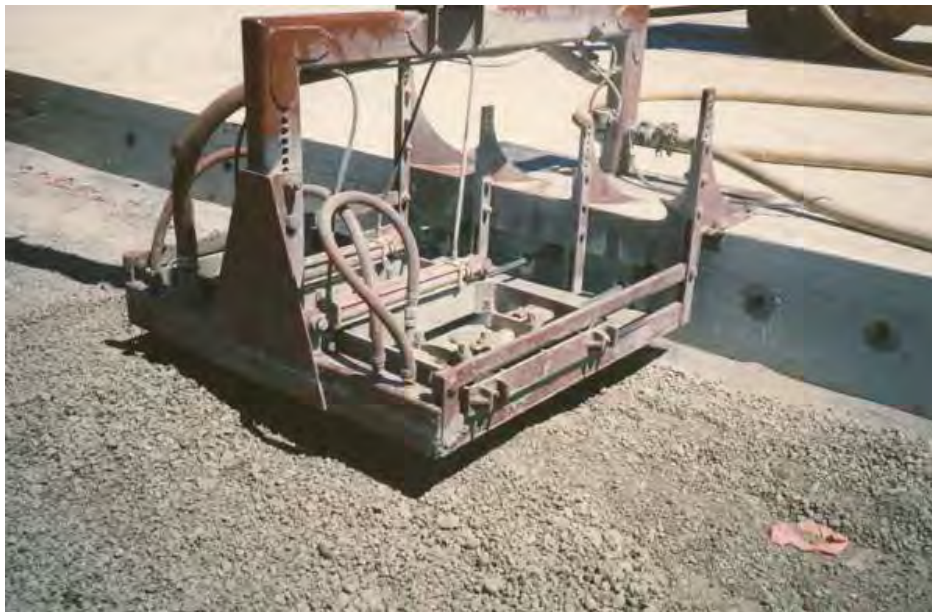
Figure 4-56 Drilling Construction Joint Dowel Holes
