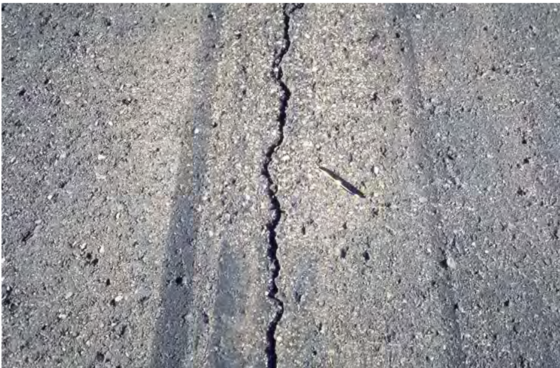
Figure 3-18 Typical Crack that should be Sealed Prior to Overlay
