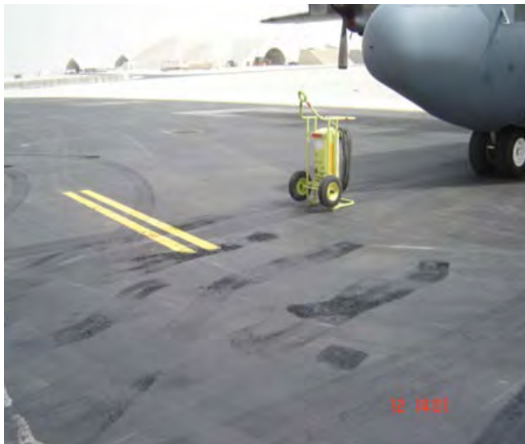
Figure 3-55 Surface Distortion
