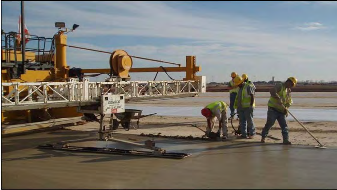
Figure 4-102 Longitudinal Float Behind Slipform Paver
