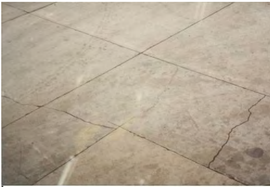
Figure 4-132 Cracks Induced by Partial Panel Replacement
