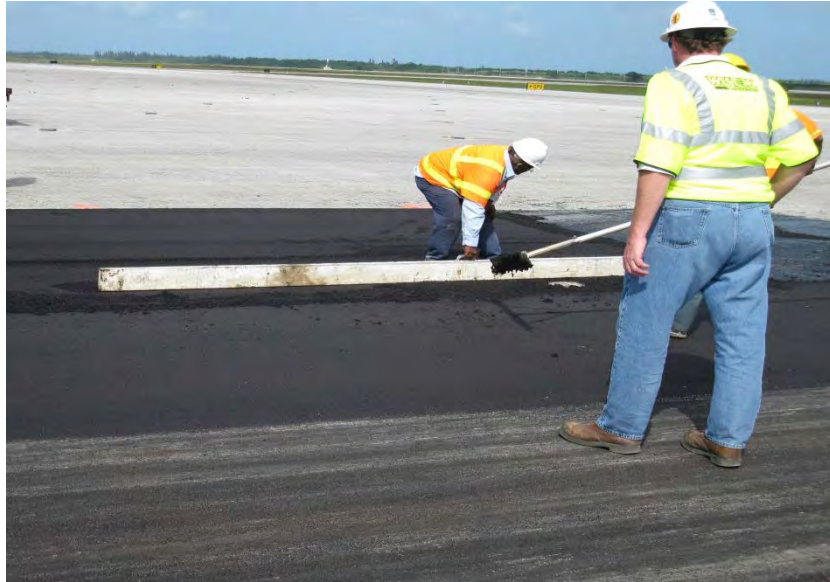
Figure 3-51 Using Straightedge to Check Smoothness
