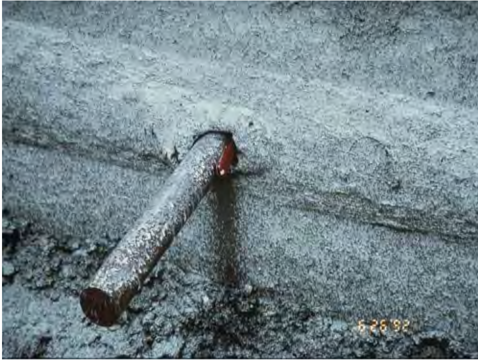
Figure 4-54 Voids around an Inserted Dowel
