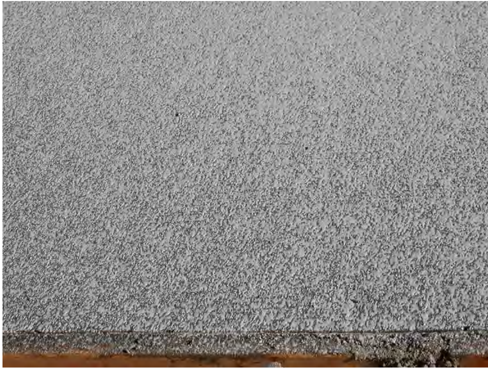
Figure 4-119 Excessive Rain Damage
