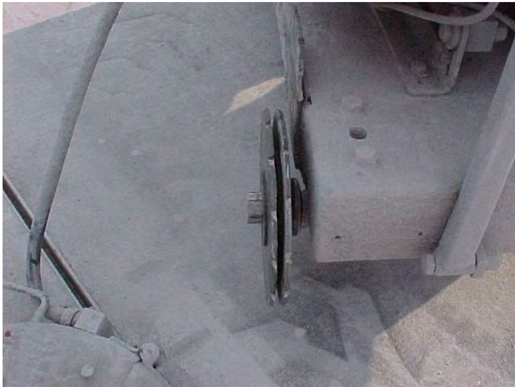
Figure 4-148 Blades used to Chamfer Joint Reservoirs
