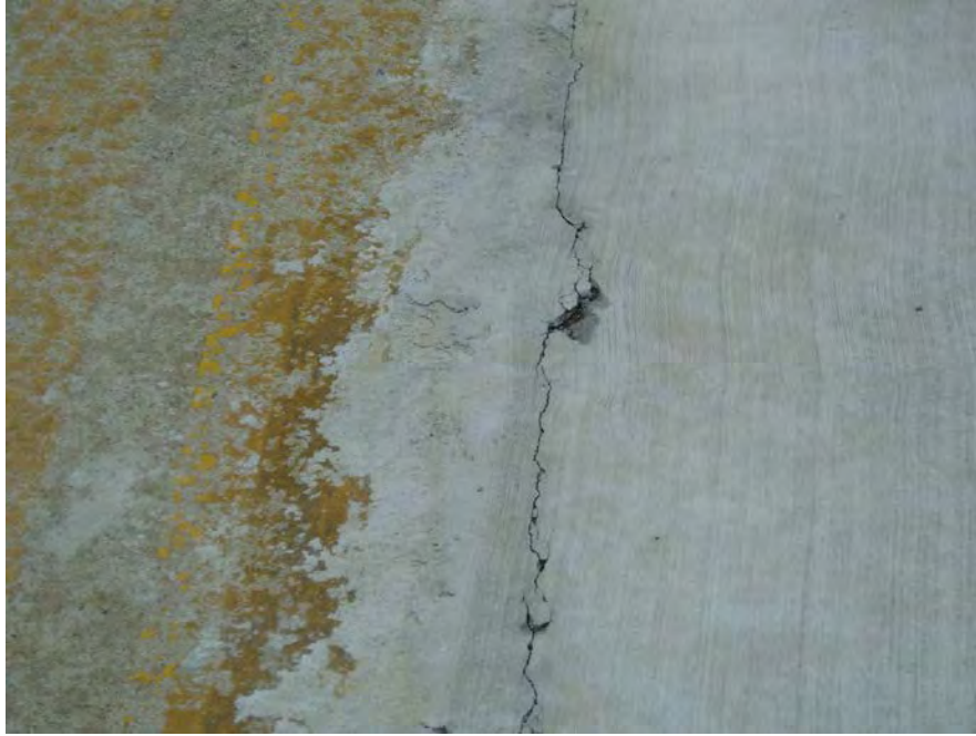
Figure 4-147 Non-Uniform Joint Cut Width
