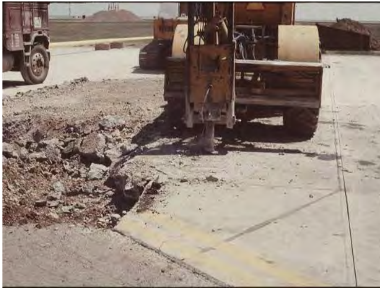
Figure 4-27 Under-breaking from Incorrect Removal Techniques
