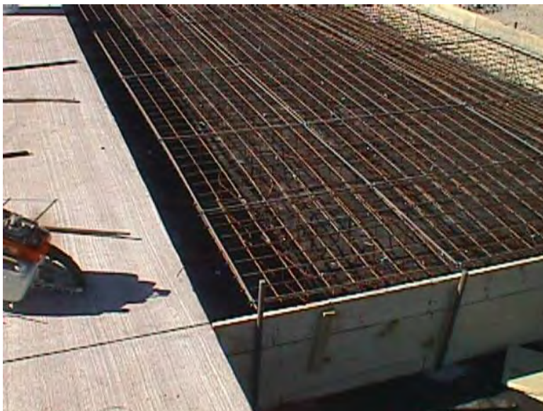
Figure 4-36 Reinforcement Steel for Odd (or Irregular)-Shaped Panels
