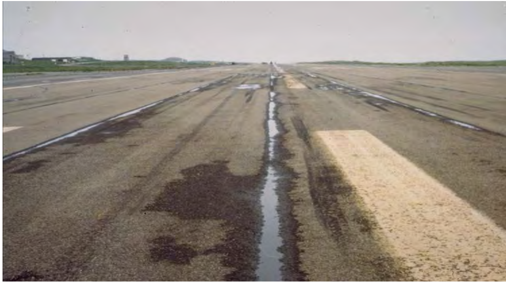
Figure 3-43 Raveling in Longitudinal Joint due to Poor Compaction
