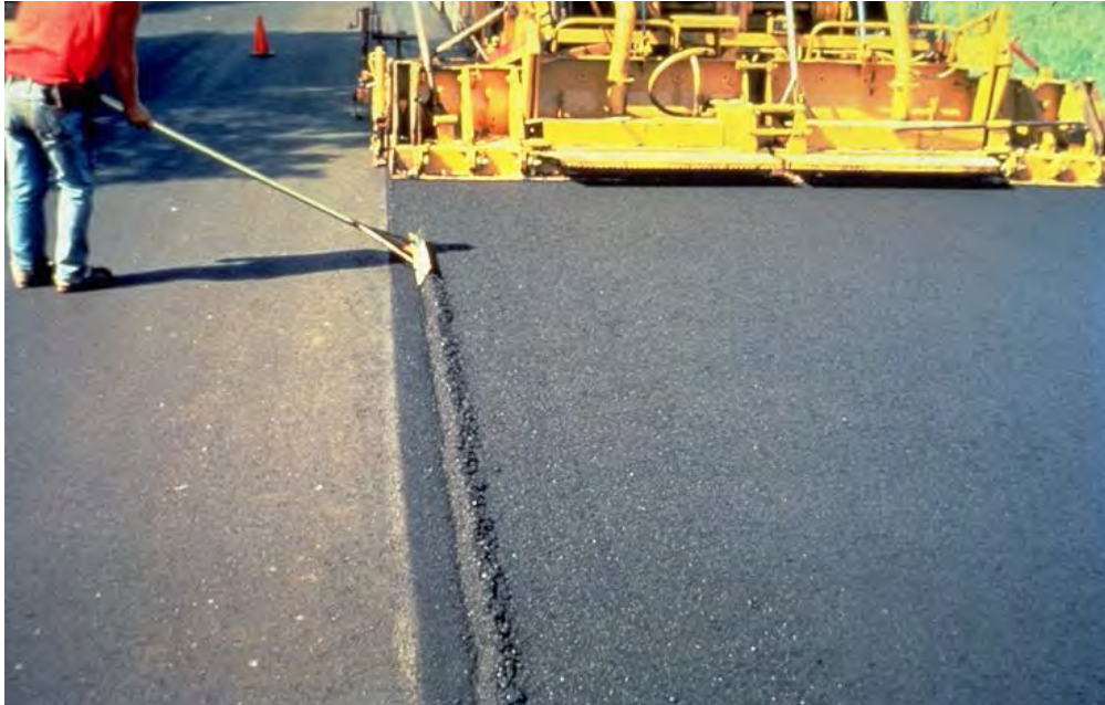
Figure 3-35 Proper way to Rake Joint
