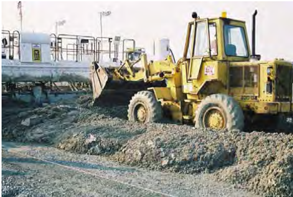
Figure 4-74 Front End Loader Distributing Concrete on Aggregate Base Course
