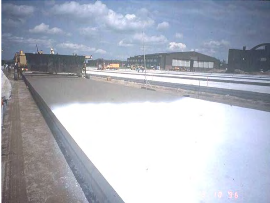
Figure 4-114 Good Application With Overlapping Spray and Windscreens
