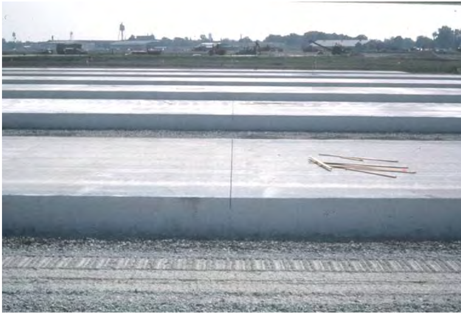
Figure 4-136 Lined Up Transverse Joints Across Pilot Lanes
