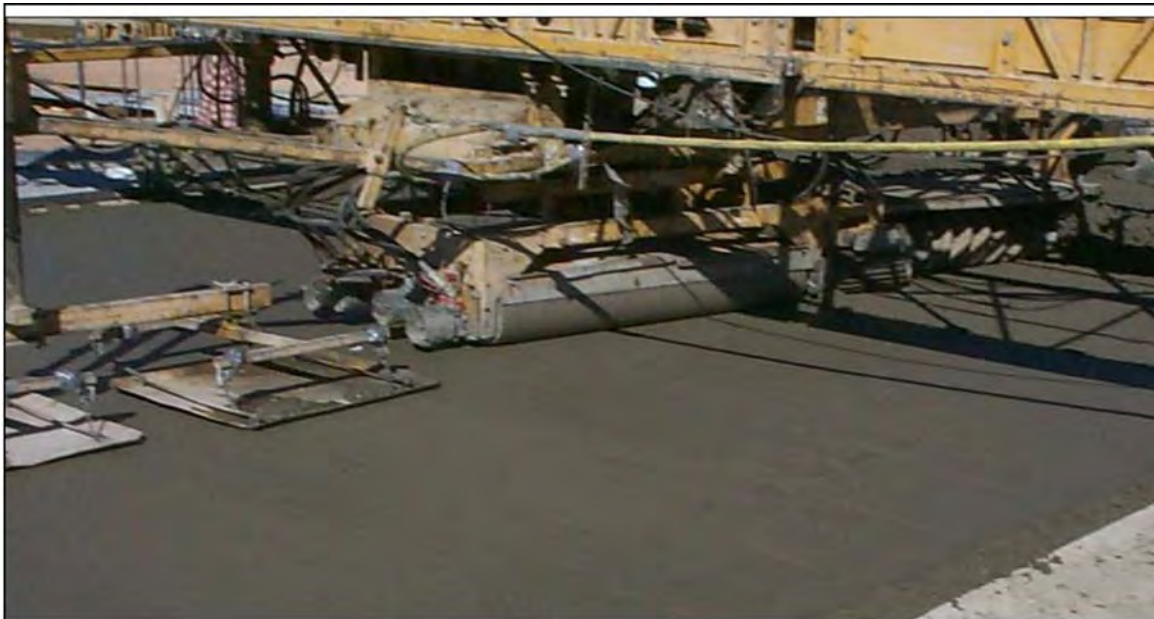
Figure 4-103 Float Pans Behind Truss-Mounted Paver
