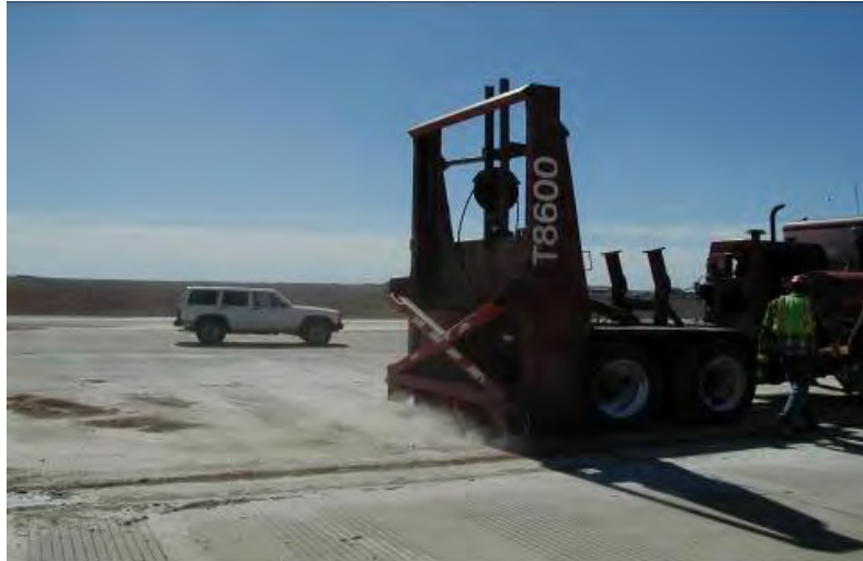
Figure 4-29 Demolition With No Protection of Adjacent Concrete
