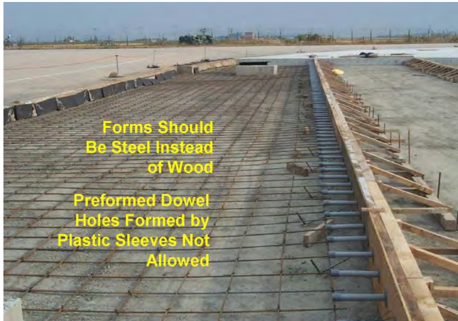
Figure 4-52 Plastic Sleeves on Wood Forms
