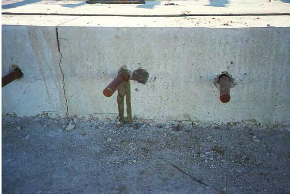
Figure 4-61 Grout Leakage with No Retention Ring
