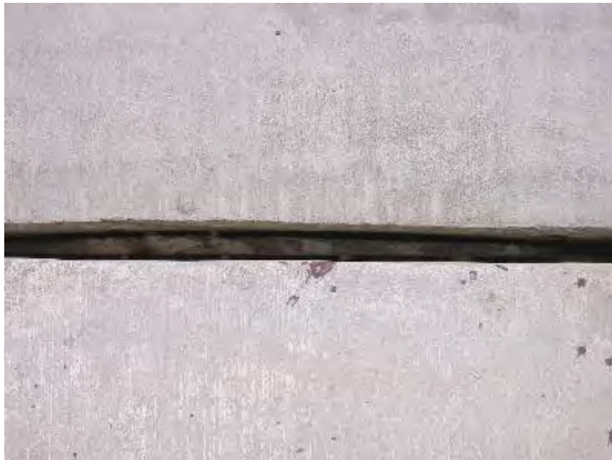
Figure 4-147 Non-Uniform Joint Cut Width
