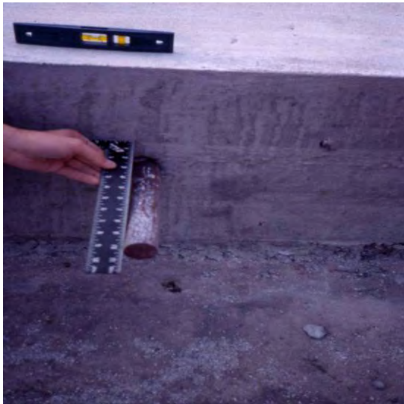
Photo 4-66 Checking Dowel for Horizontal Alignment
