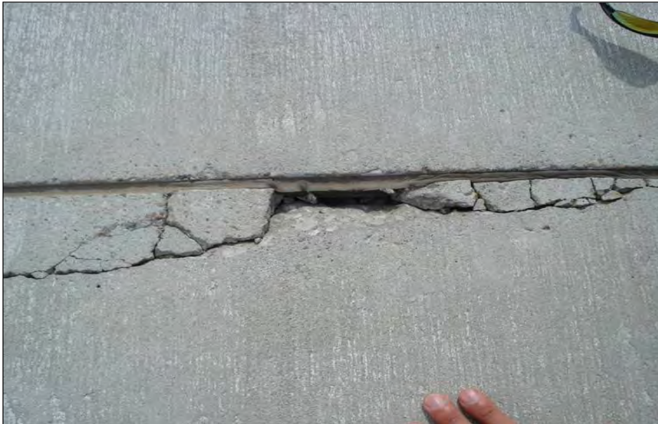
Figure 4-160 Spalls along Joint Line
