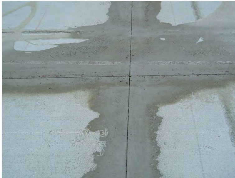
Figure 4-140 Cuttings Not Removed
