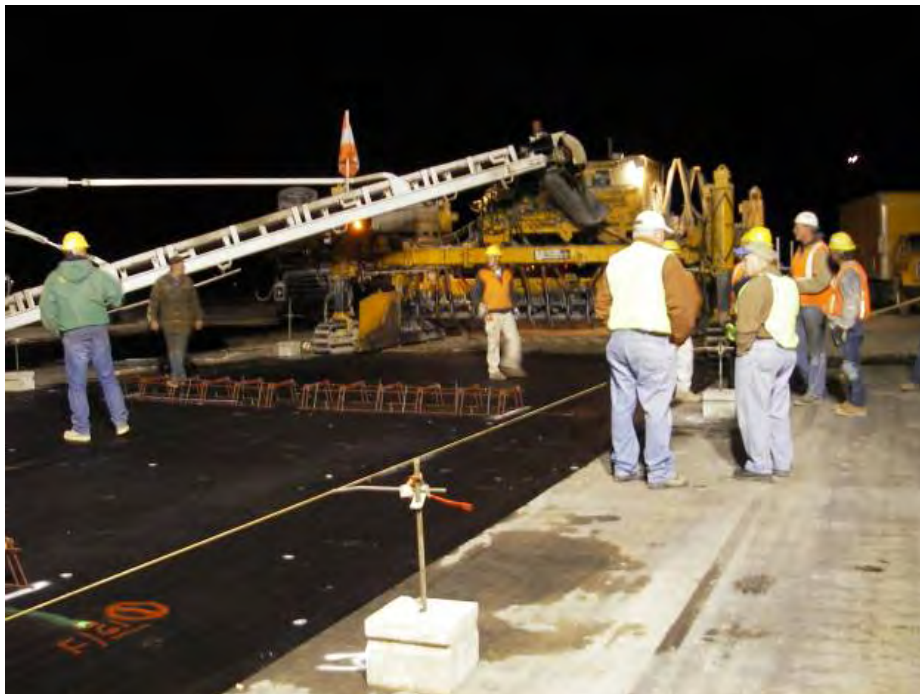
Figure 4-76 Dropping Concrete in Excess of Five Feet
