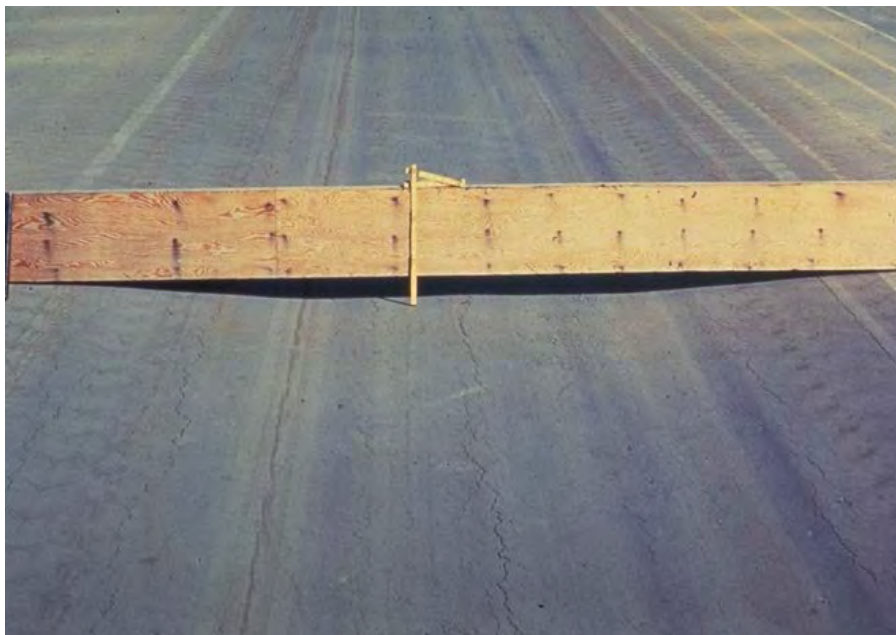
Figure 3-53 Structural Rutting Caused by Problems Underneath Asphalt Mixture
