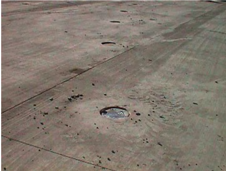
Figure 4-133 Light Cans Properly Located With the Joints
