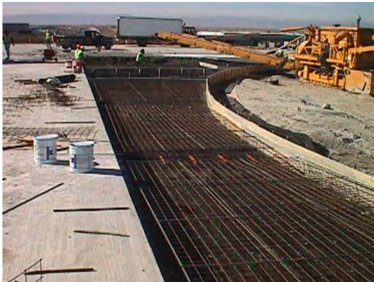
Figure 4-36 Reinforcement Steel for Odd (or Irregular)-Shaped Panels
