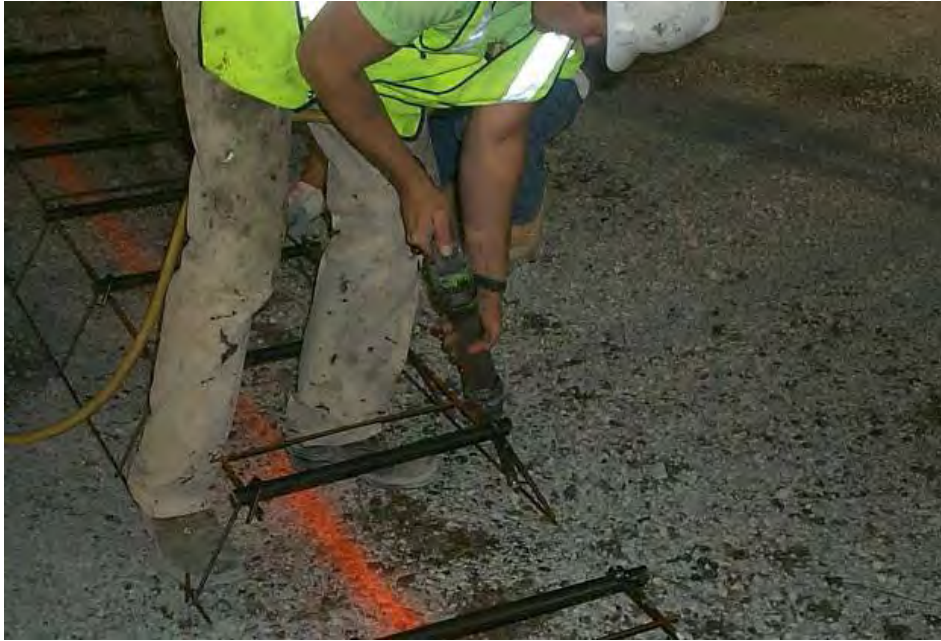
Figure 4-47 Securing Dowel Baskets
