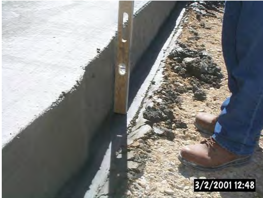
Figure 4-129 Poor Quality Construction Joint
