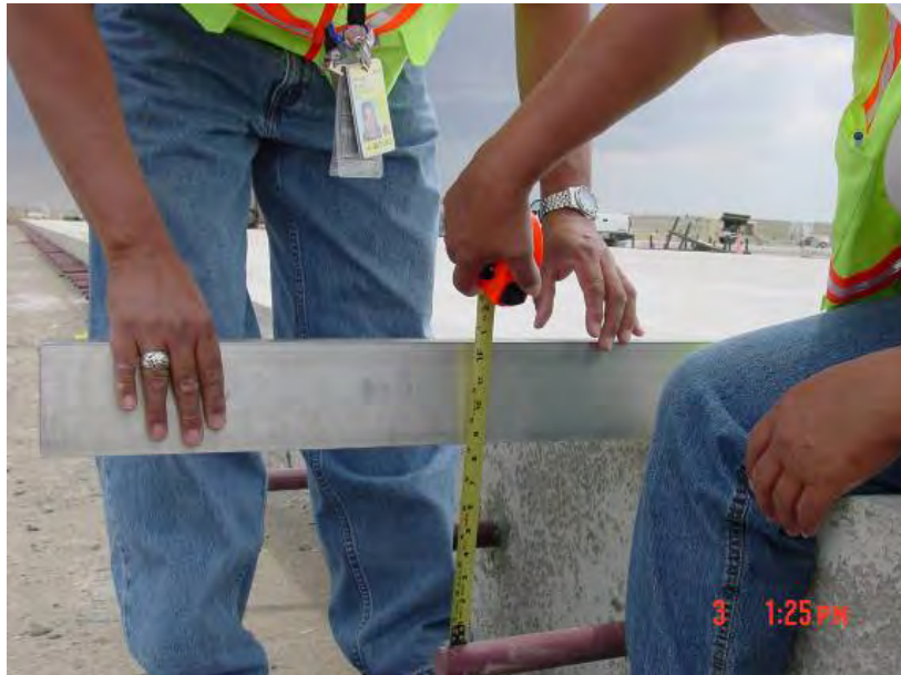
Figure 4-67 Checking Dowel for Vertical Alignment
