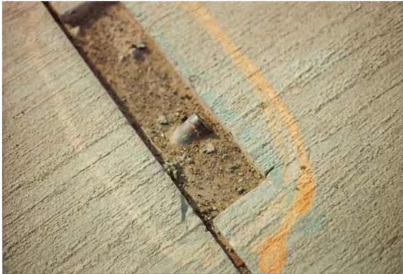
Figure 4-50 Misaligned Contract Joint Dowels
