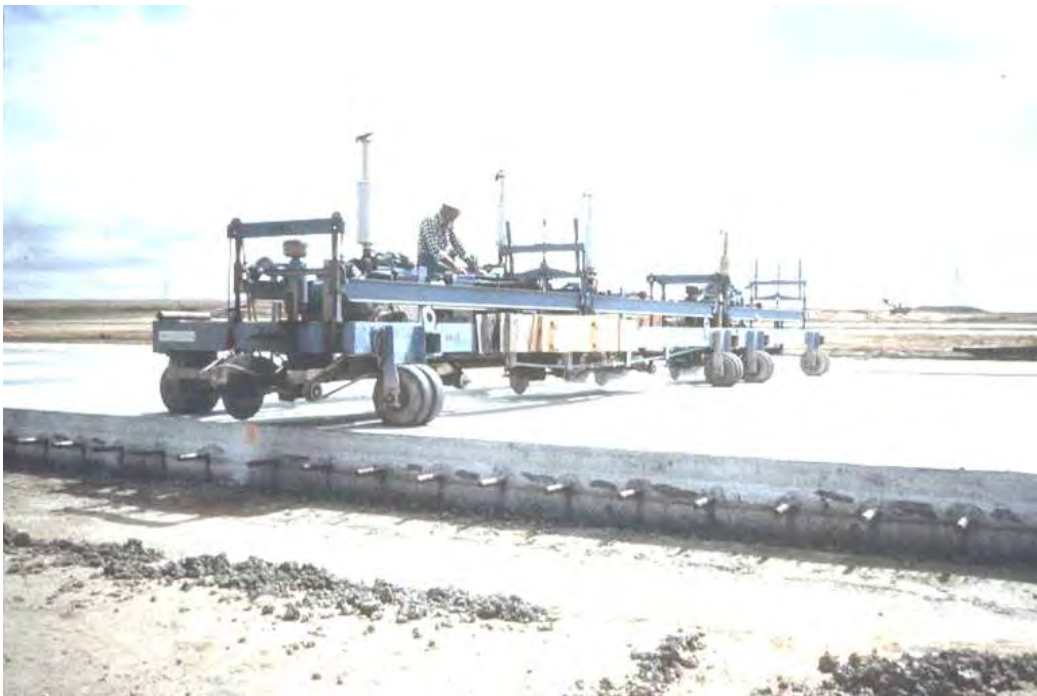
Figure 4-142 Saw Cutting Machine With Multiple Blades
