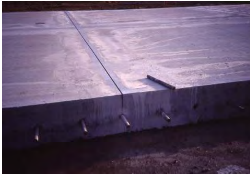
Figure 4-46 Dowel Located on a Contraction Joint.
