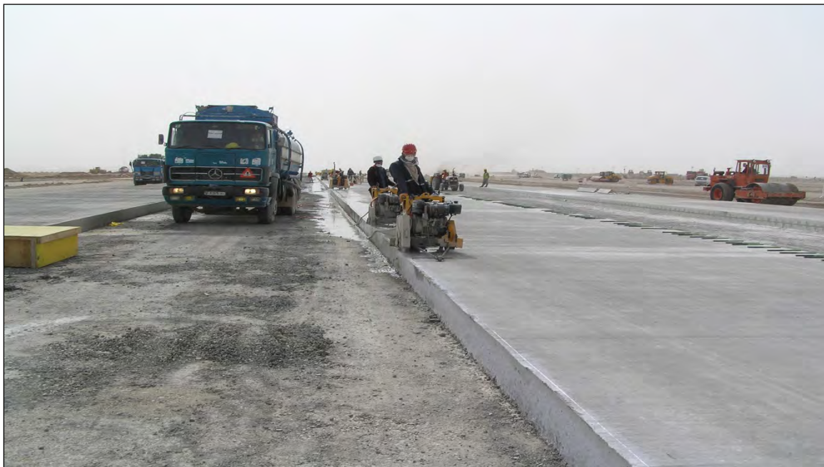
Figure 4-158 Saw Cutting Vertical Joint Face
