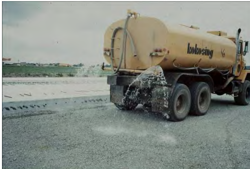
Figure 4-19 Dampening the Base Course
