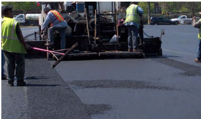
Figure 3-36 Texture Difference Under Screed on Both Sides of Paver (Paver Extensions)
