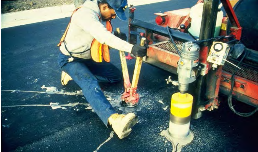
Figure 3-48 Cutting Cores for Density Testing
