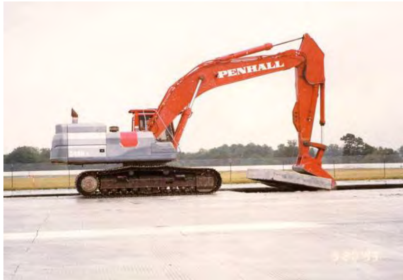
Figure 4-30 Removal of Saw-Cut Pavement Pieces
