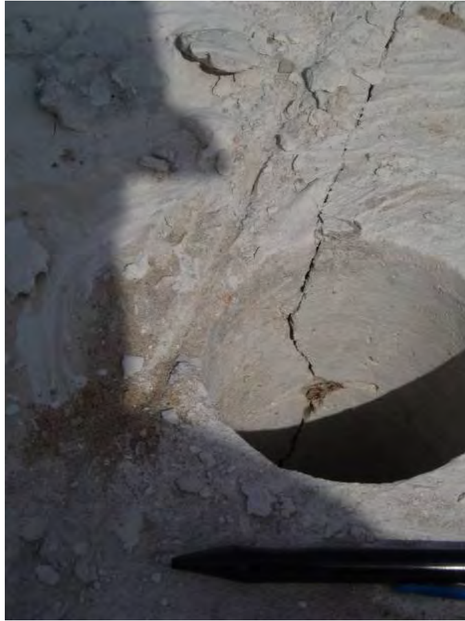
Figure 4-40 Cracked Panels from Misplaced Reinforcement Steel
