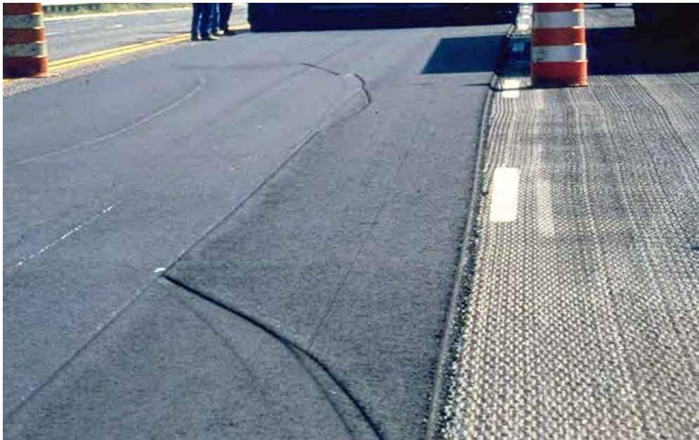
Figure 3-47 Excessive Roller Marks
