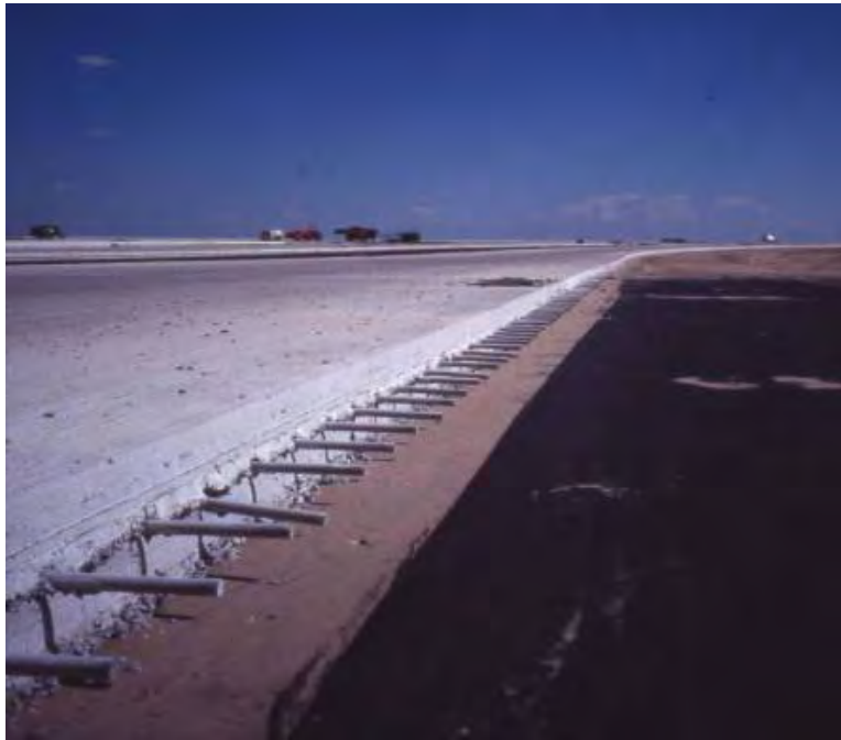
Figure 4-55 Alignments of Inserted Dowels
