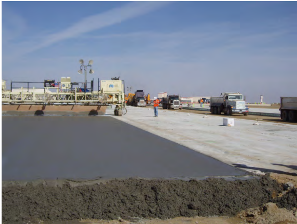
Figure 4-68 Backup of Trucks at Paving Site
