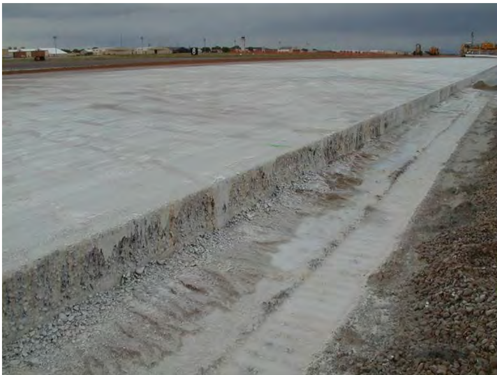
Figure 4-119 Excessive Rain Damage
