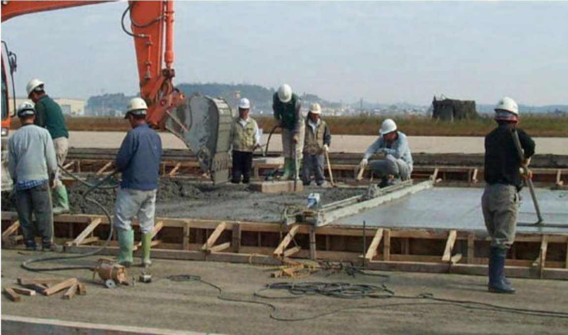
Figure 4-95 Hand-Held, Pneumatic Vibrator
