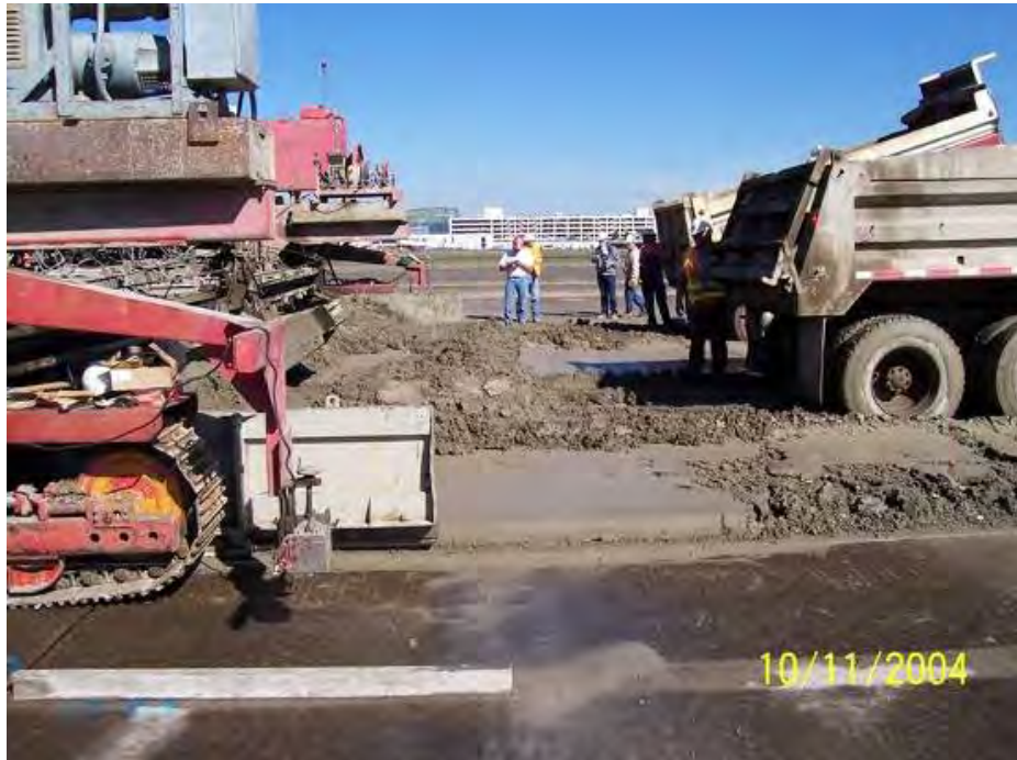
Figure 4-77 Backing Trucks Down Paving Lane
