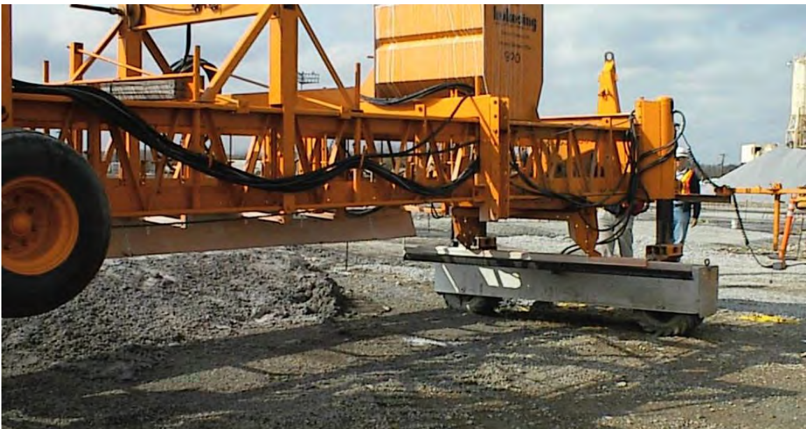
Figure 4-110 Broom Texturing Equipment
