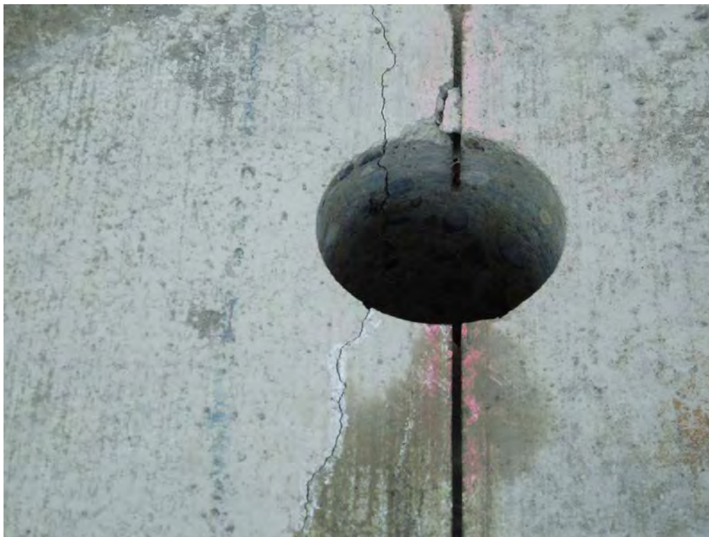
Figure 4-145 Core to Verify Depth of Crack
