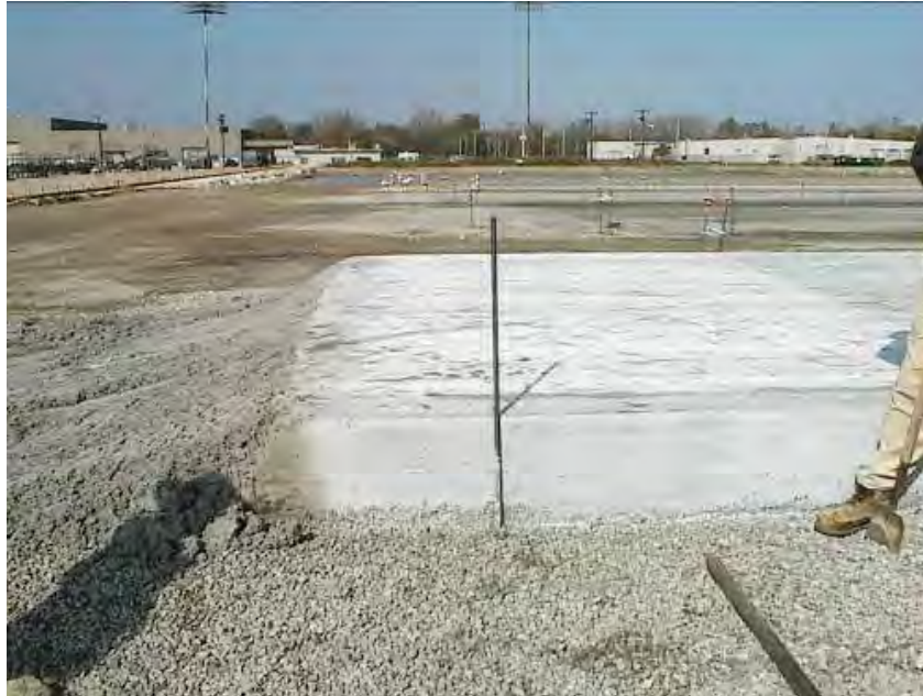
Figure 4-128 Paving Through and Sawing Off End
