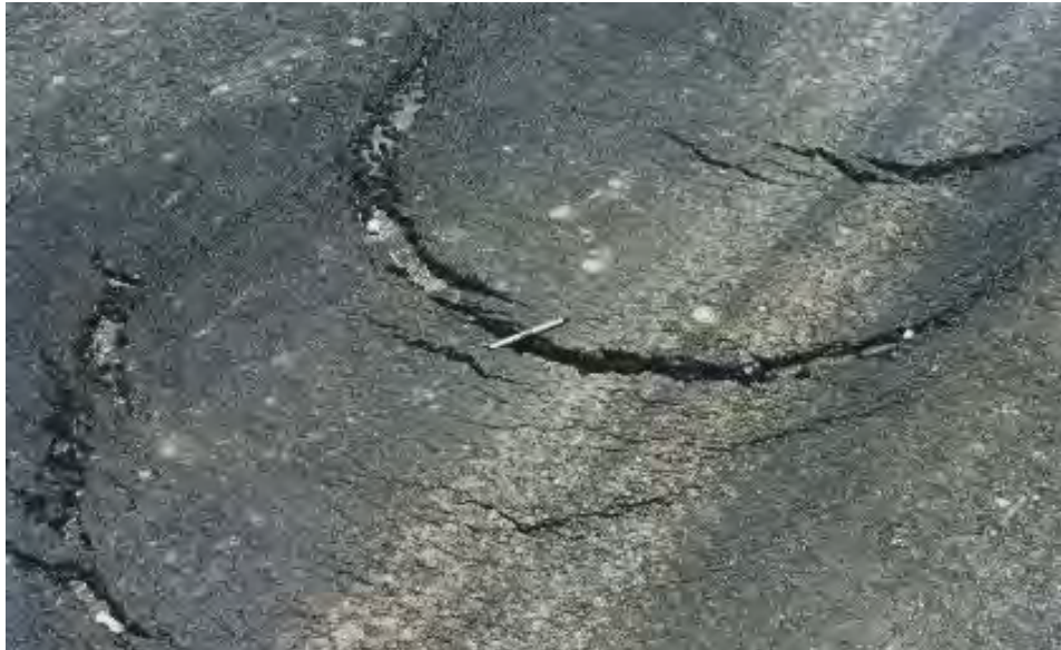
Figure 3-58 Slippage of Asphalt Mixture over Underlying Layer
