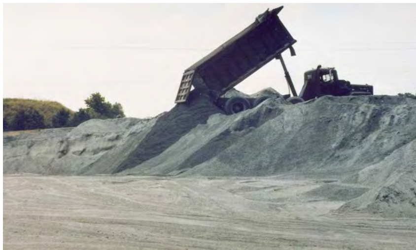
Figure 3-6 Improper Addition of Material to a Stockpile
