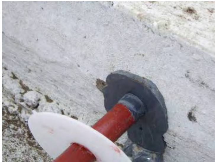
Figure 4-63 Dowel with Retention Ring
