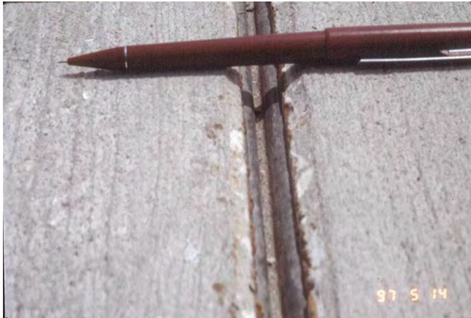
Figure 4-149 Chamfered and Sealed Joint
