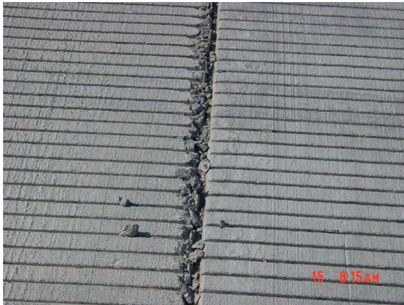
Figure 4-121 Spall Damage
