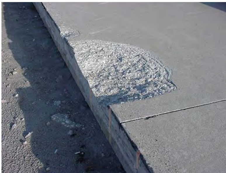
Figure 4-121 Spall Damage
