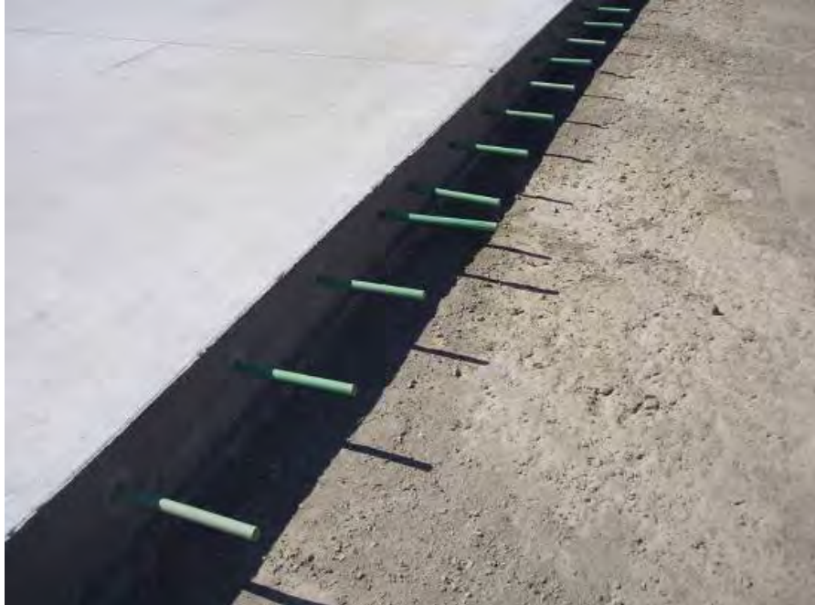
Photo 4-65 Misaligned Dowels
