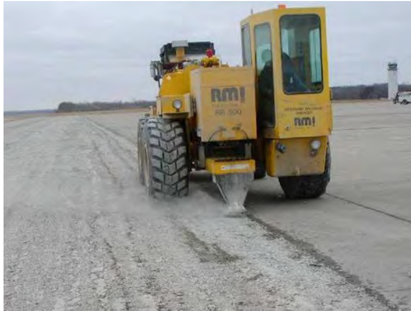
Figure 4-32 Resonant Pavement Demolition
