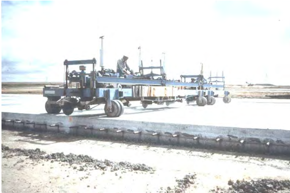
Figure 4-116 Poor Application of Curing Compound Vertical Joint
