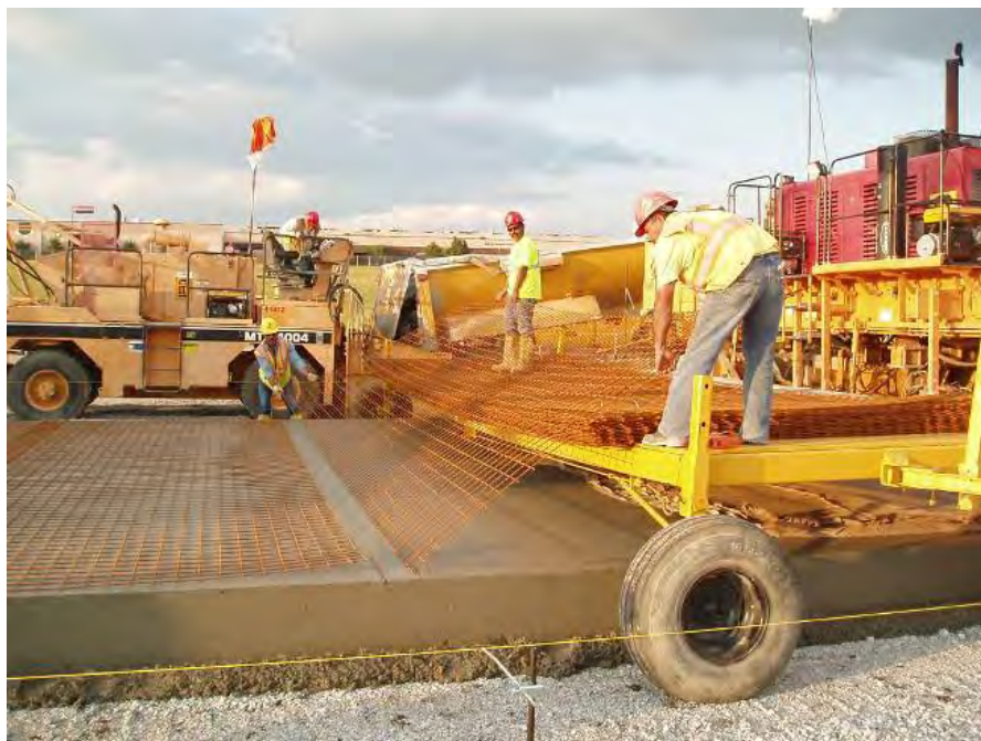
Figure 4-39 Gap in Reinforcing steel at Contraction Joint
